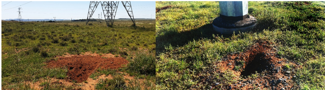
Figure 3: Active burrows in close proximity to power line infrastructure, indicating that the presence of these structures did not deter burrowing animals from the site. Springhare potentially take advantage of the disturbed soil and short grasses surrounding the pylons.
