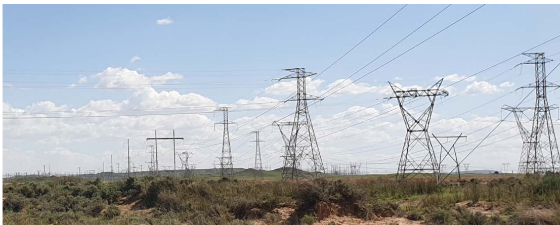
Figure 3: Multiple electricity transmission lines exist converging on the Hydra Main Transmission Substation.
