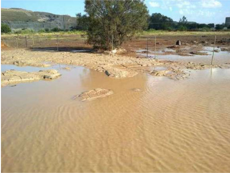
On the 30th of October 2012 a containment wall collapsed causing toxic and radioactive contamination of farmland
