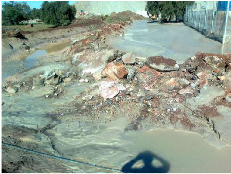
Midway Dam, containing contaminated process water overflowing its walls.
