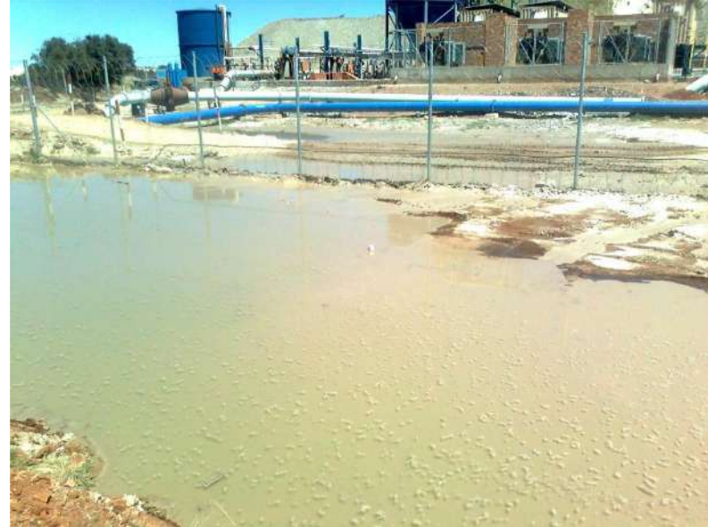
Toxic and radioactive spillages from Pump Station No 2.
