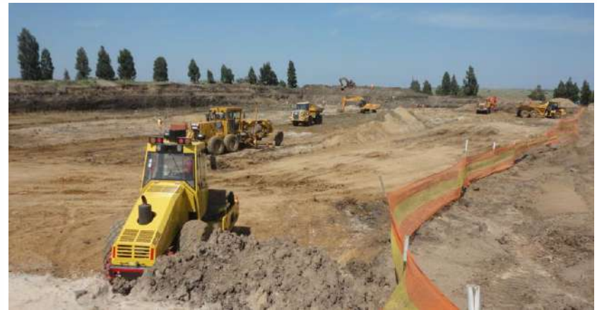
Additional water containment dam - Kareerand
