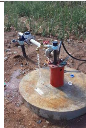
Interception boreholes Kareerand
