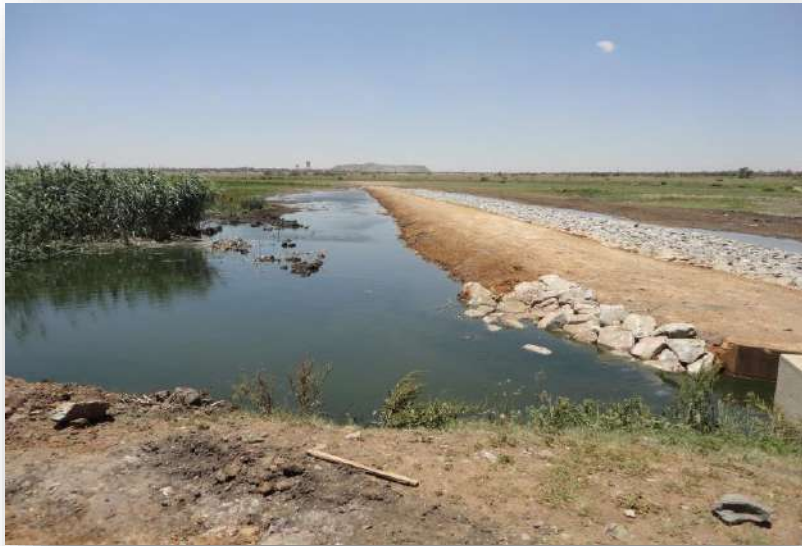
Downstream containment – Koekemoer Spruit
