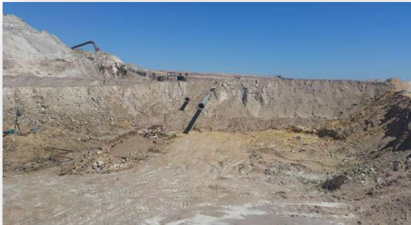
Reclamation Site - Containment
