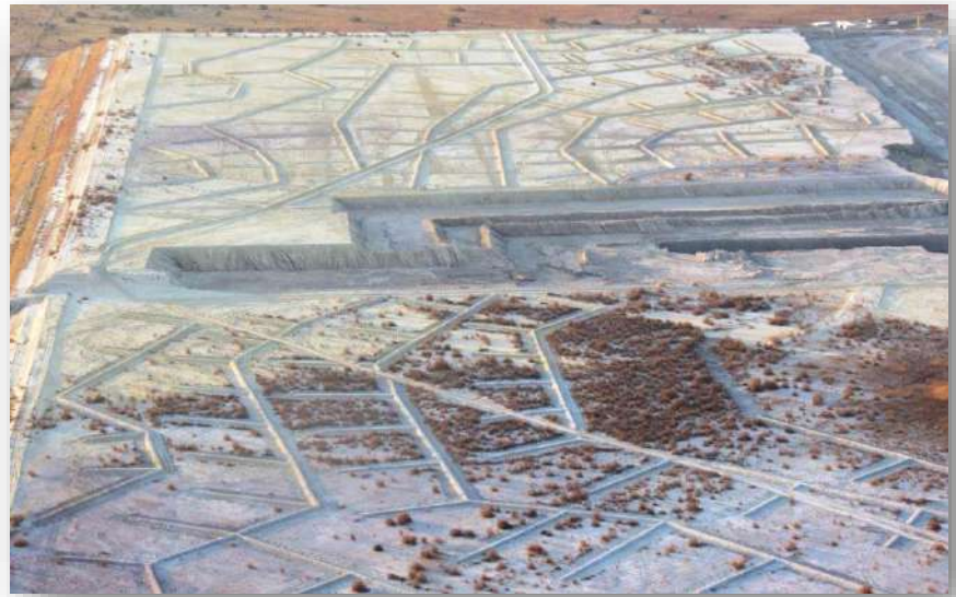
Containment paddocks – TSF being reclaimed
