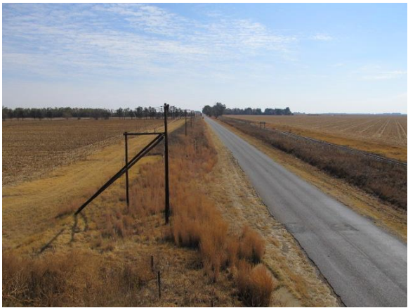
A photograph of the railroad and Krige Street towards the south west of the site.
