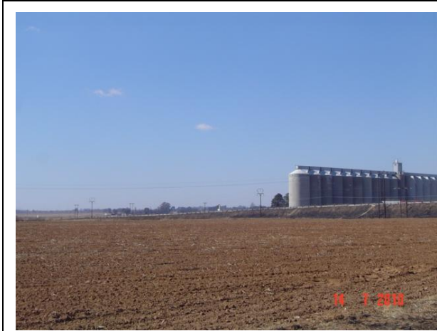
A photograph taken from the railroad towards the site.
