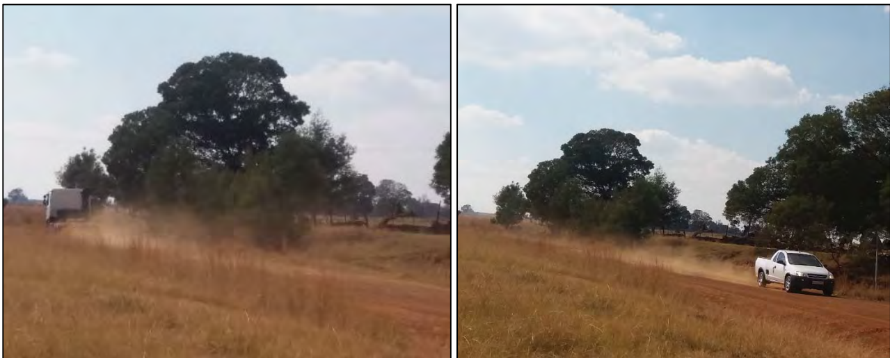
Figure 11: Dust generated on D648 by an heavy (left) and light (right) motor vehicles (Golder, 2016)
