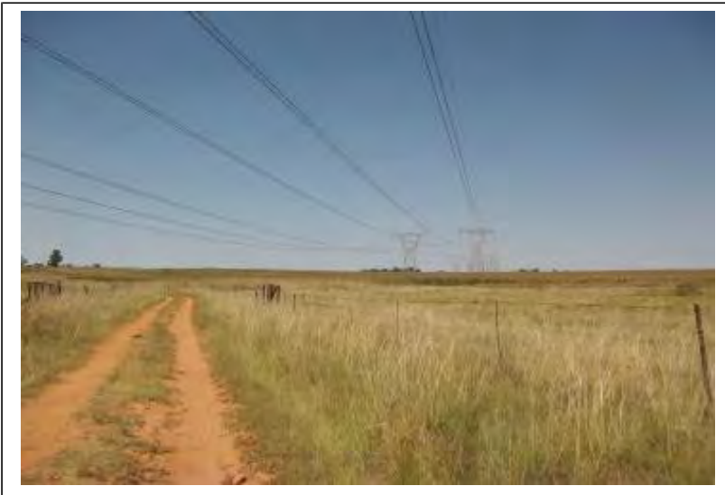
Figure 59: Preferred alternative route F runs along Eskom's existing 400 kV power lines
