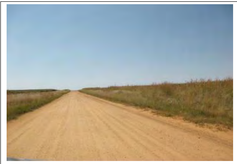
Figure 60: Short stretches of existing roads such as D1574, D685, D1048 and D684 cross the project area
