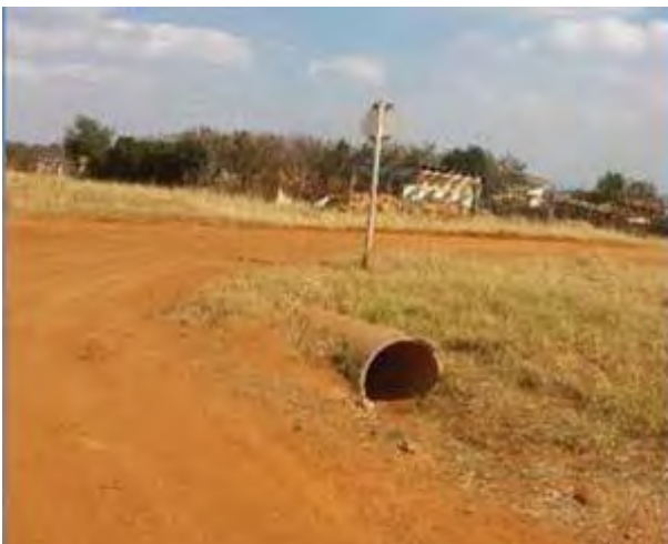
Figure 54: Culvert installed at Sikhululiwe Village entrance
