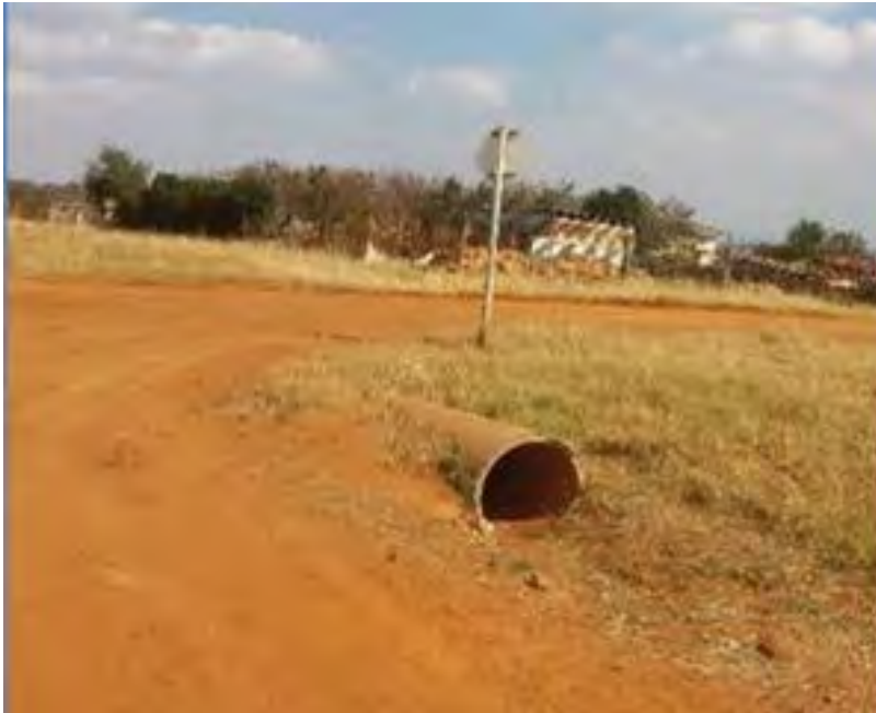
Figure 65: Culvert installed at Sikhululiwe Village entrance
