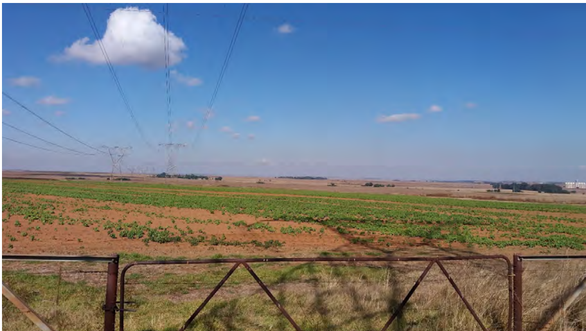
Figure 20: View of the Alternative F route option taken from its proposed beginning just off the D684 road
