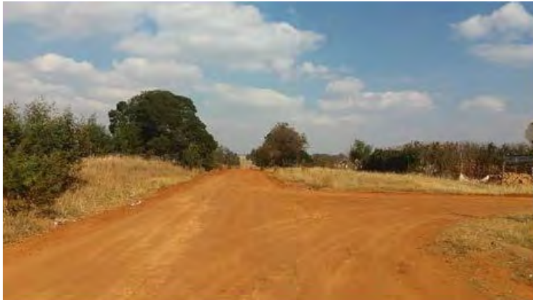
Figure 61: Southerly view of D648 from survey point
