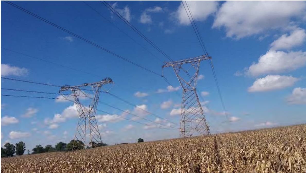
Figure 20: View of the Alternative F route option – photo taken from the D1048 road
