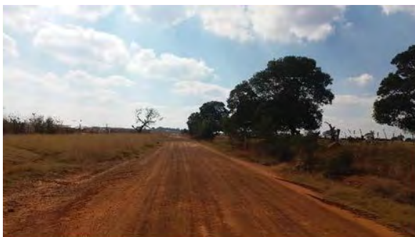
Figure 60: Northerly view of D648 from survey point
