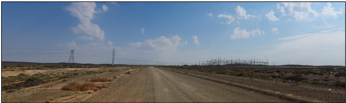
Figure 45: Existing network of powerlines converging at Helios MTS
