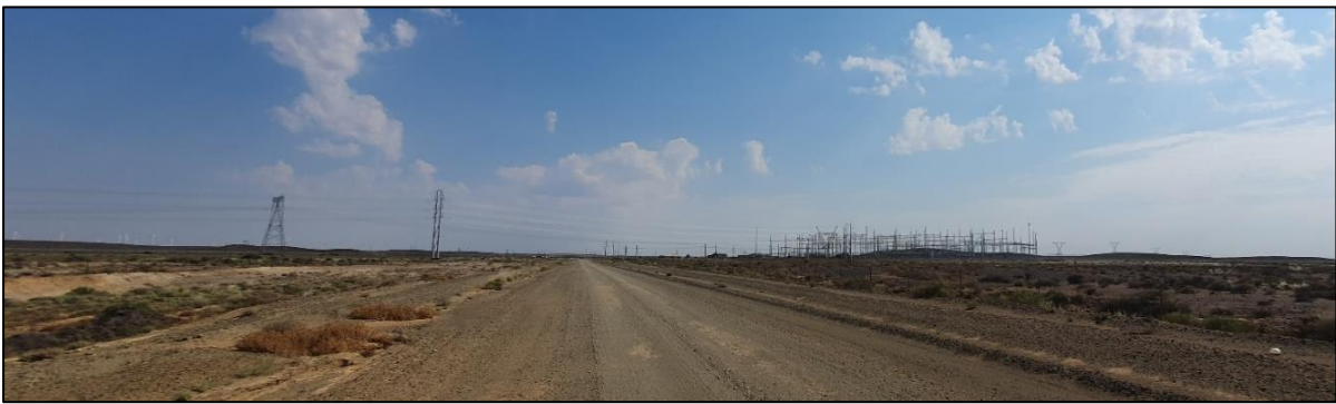
Figure 12: Existing network of powerlines converging at the Helios MTS
