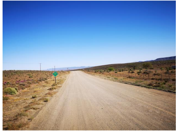
Image 5-2 Typical condition of R355
