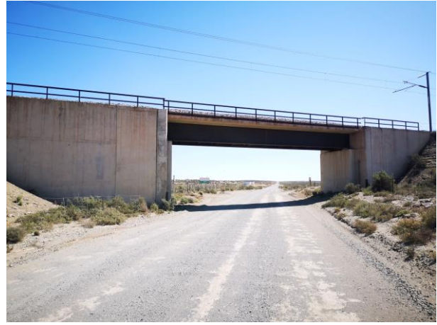
Image 5-6 Railway bridge over AP2972 before TR1
