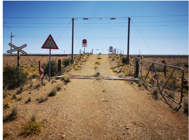
Image 5-16 SA2 from within site
