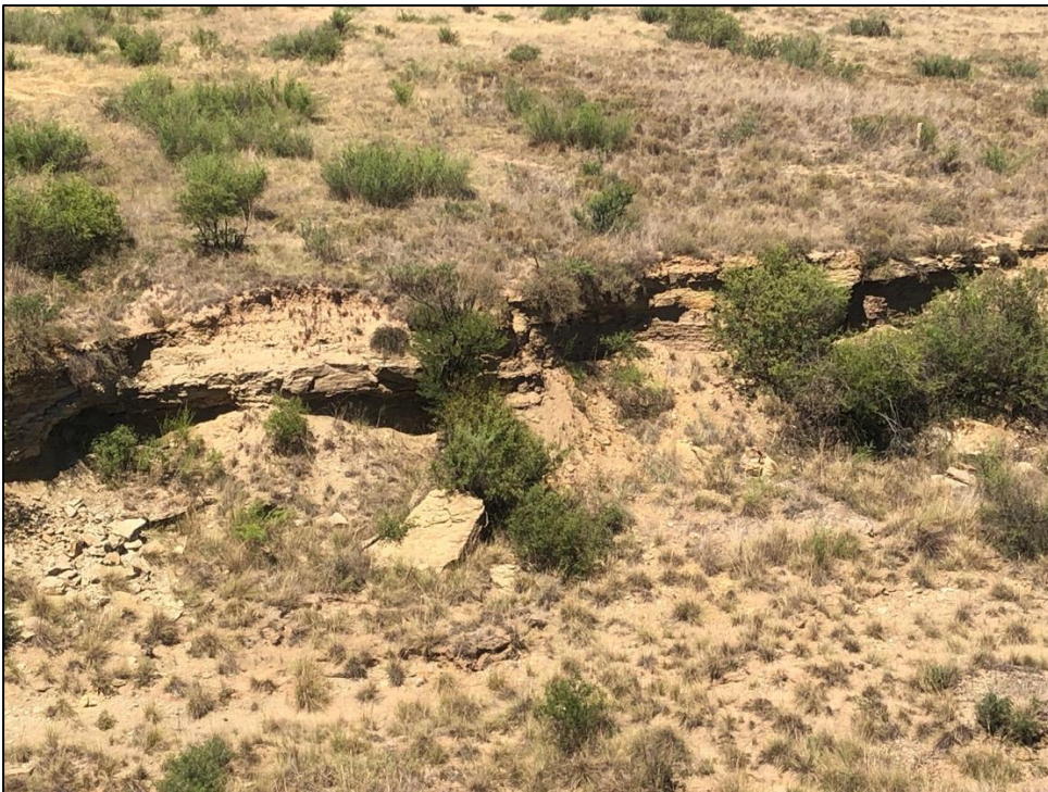
Plate 3: Several areas within the observed watercourse show signs of erosion and head cut formation, especially in the lower reaches of the systems before they join the mainstem rivers
