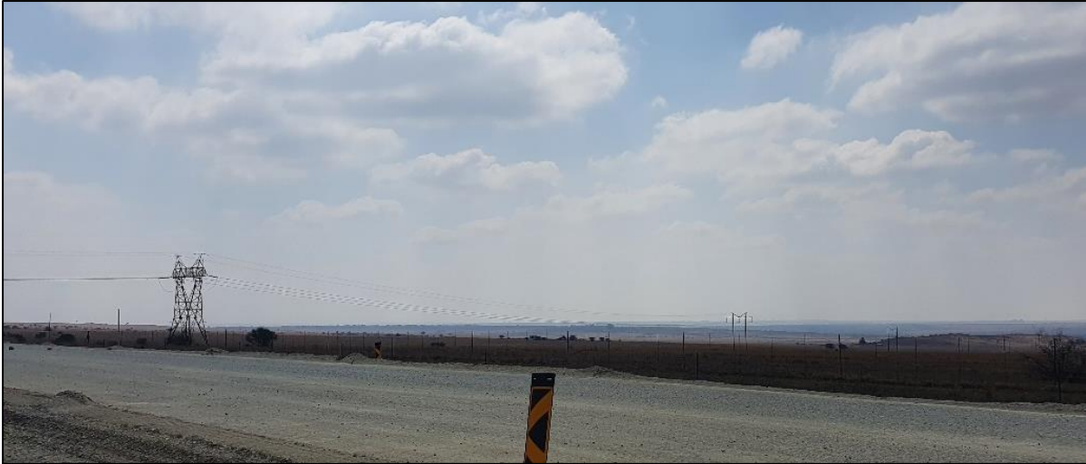
Figure 13: Existing 132kV powerline extending across the site and over the R76
