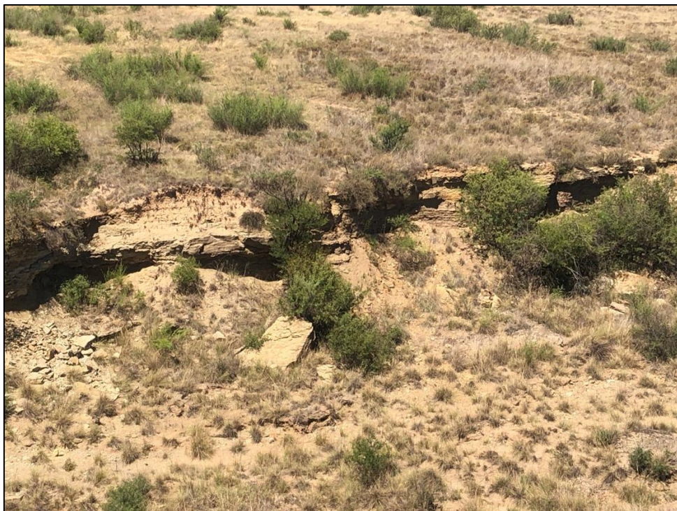
Plate 3: Several areas within the observed watercourse show signs of erosion and head cut formation, especially in the lower reaches of the systems before they join the mainstem rivers
