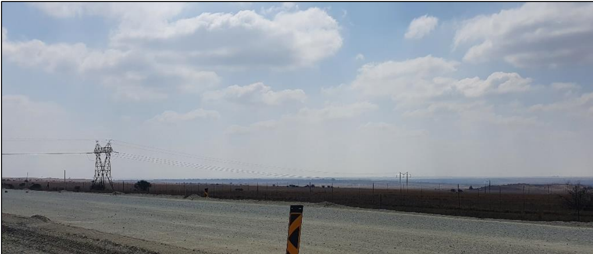
Figure 12: Existing 132kV powerline extending across the site and over the R76
