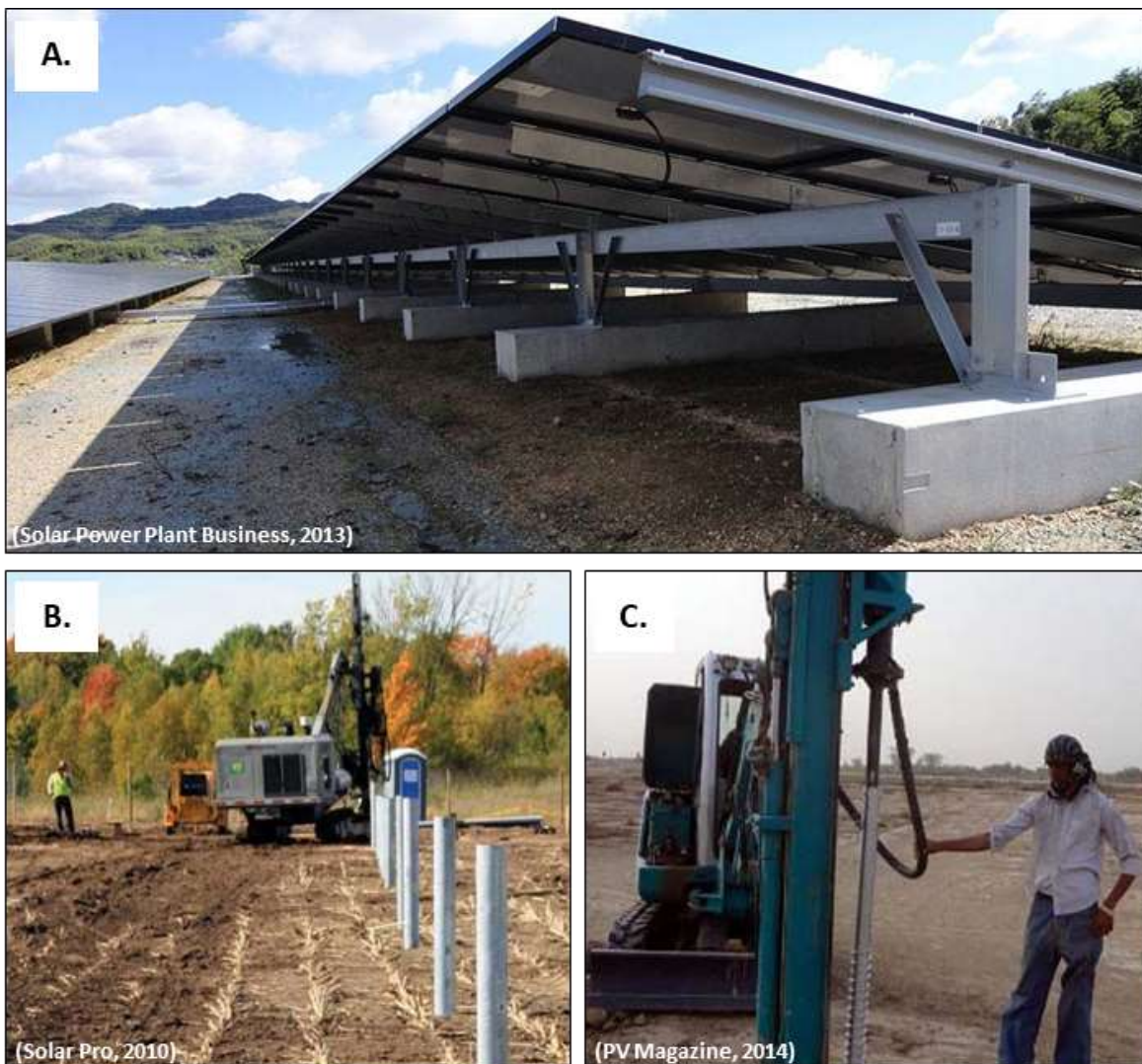
Figure 6: Mounting Structures. A) Cast Concrete Foundation. B) Driven/ Rammed Steel Pile. C) Ground / Earth Screw.
