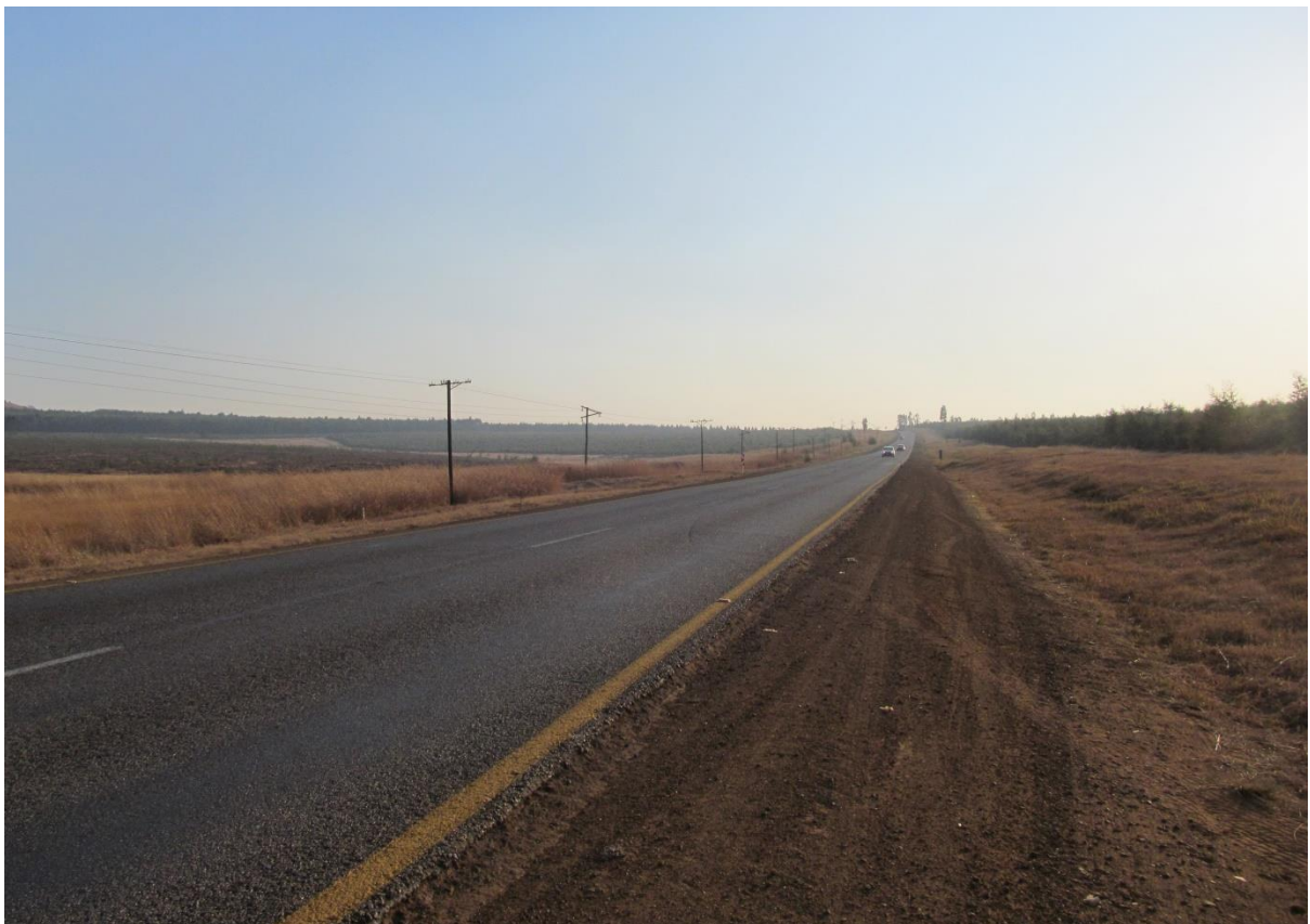
Photo 7: At km 60,0 taken to the West
