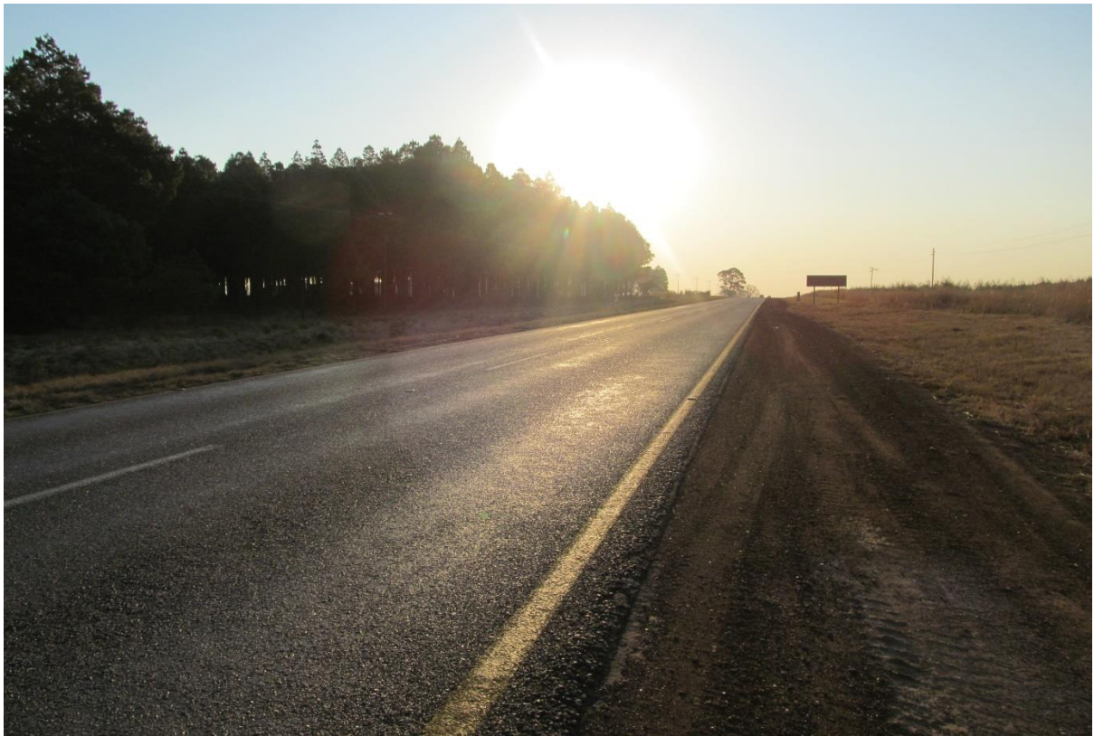
Photo 14: Taken at km 45,0 towards the North West
