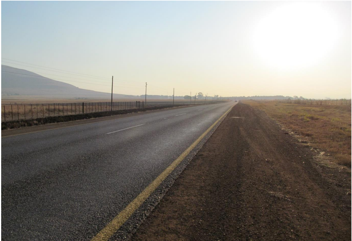
Photo 9: Taken at km 55,0 towards the West
