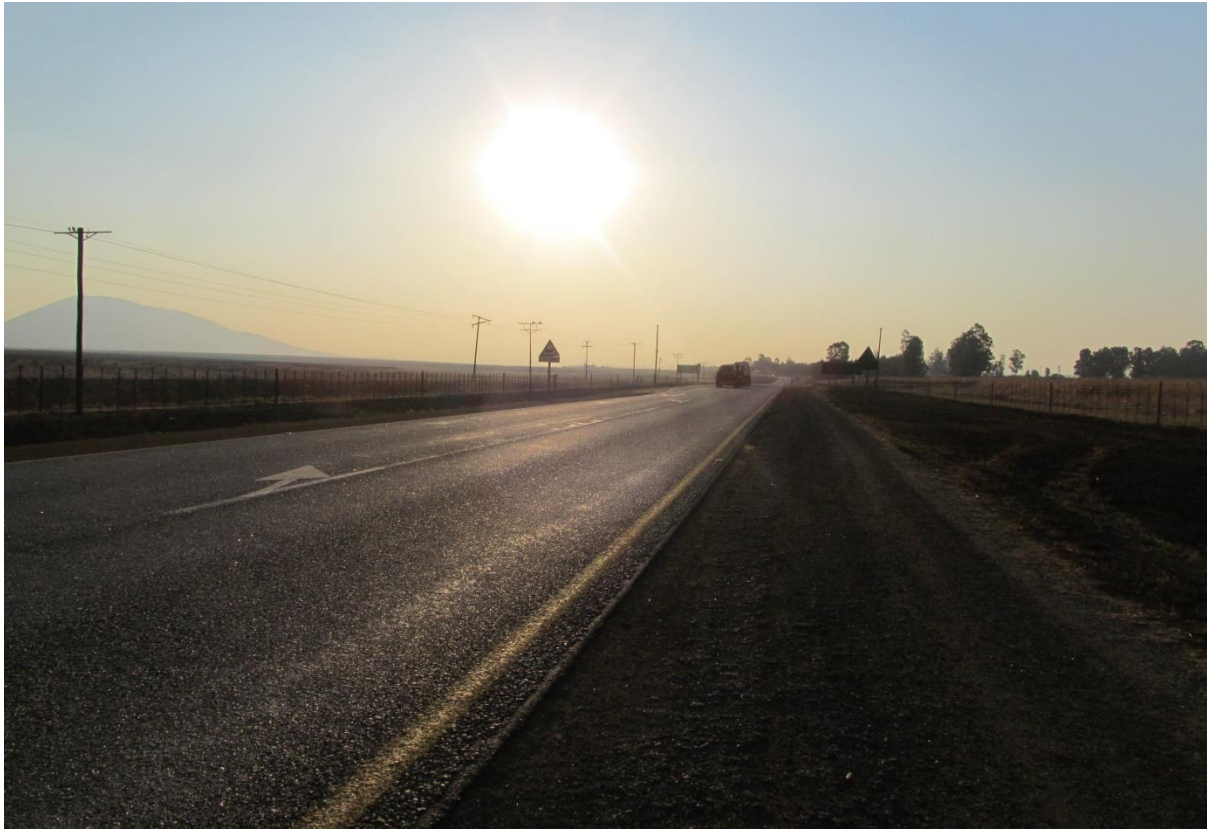
Photo 11: Taken at km 50,0 towards the West
