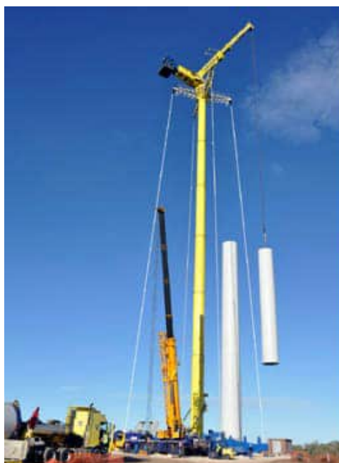
Figure 2-8:Example - Cranes at work
