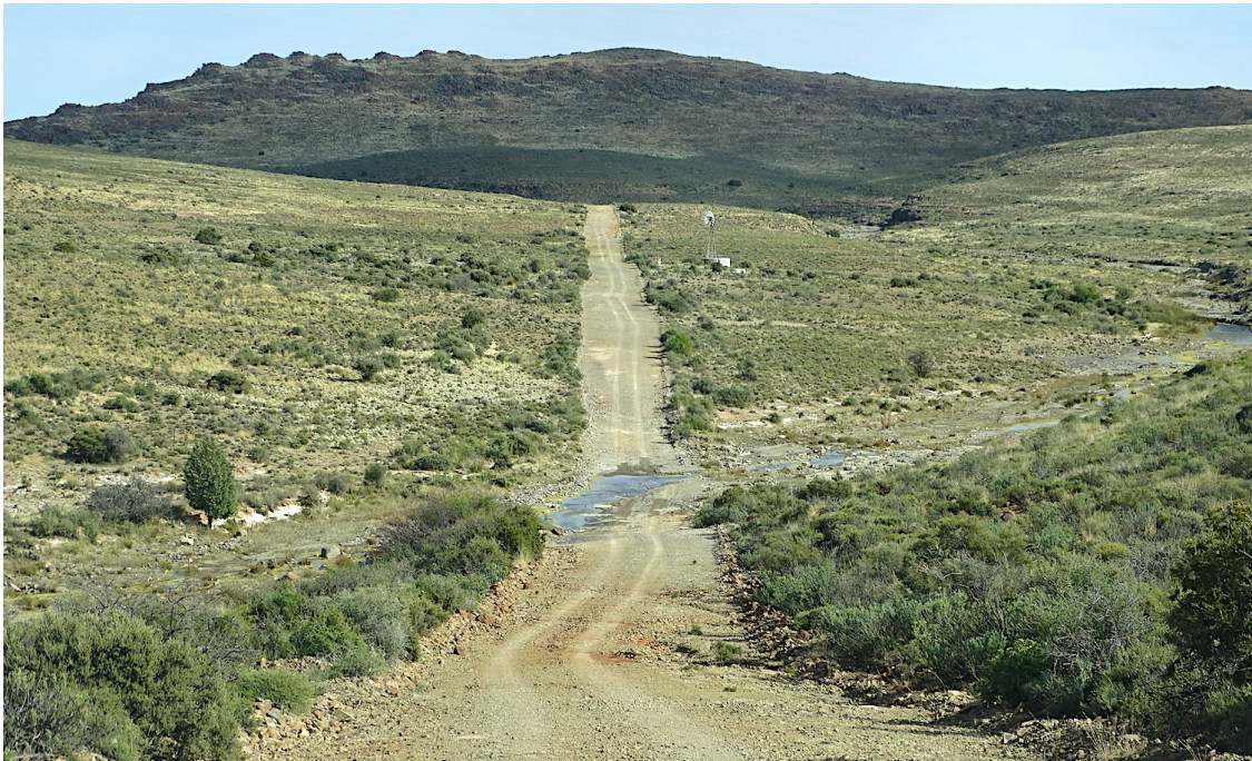
Fig. 4: Existing access road between Leeukloof and Booiskraal
