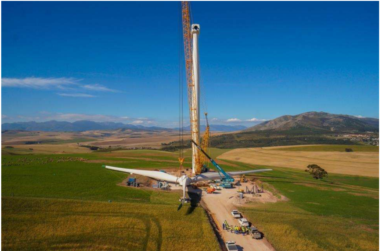
Figure 3-4: Construction of the Turbine – Preparing to lift the Rotor
