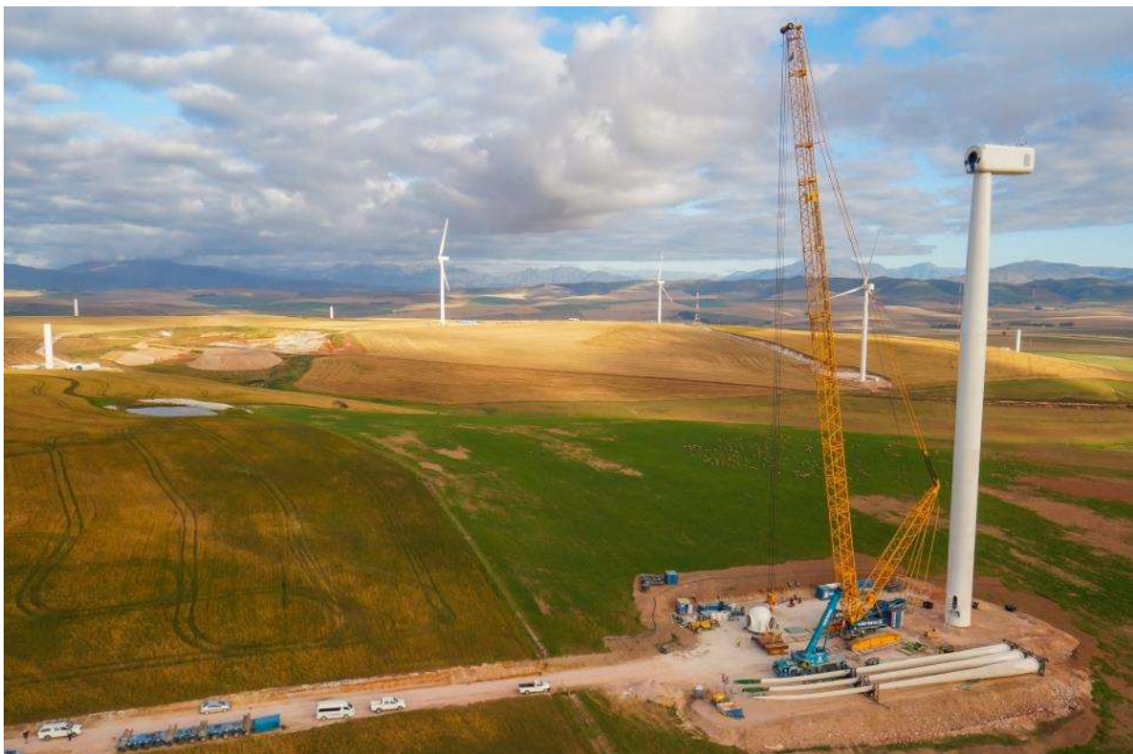
Figure 3-5: Construction of the Turbine – Lifting Equipment (i.e., Crane)
