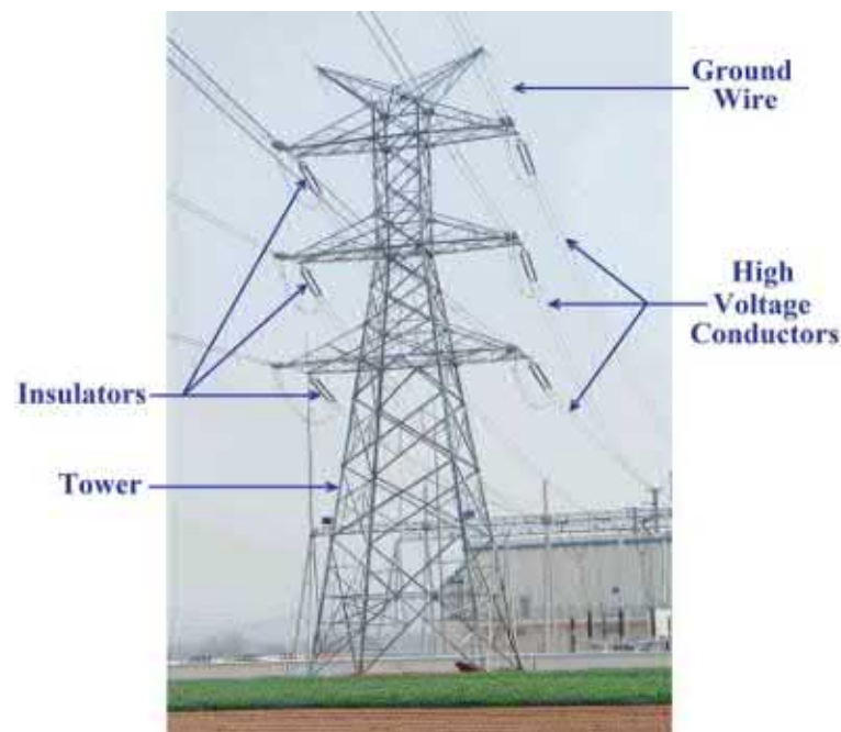
Figure 6-1: Typical High voltage Power Transmission system (Chakraborty, 2017)
