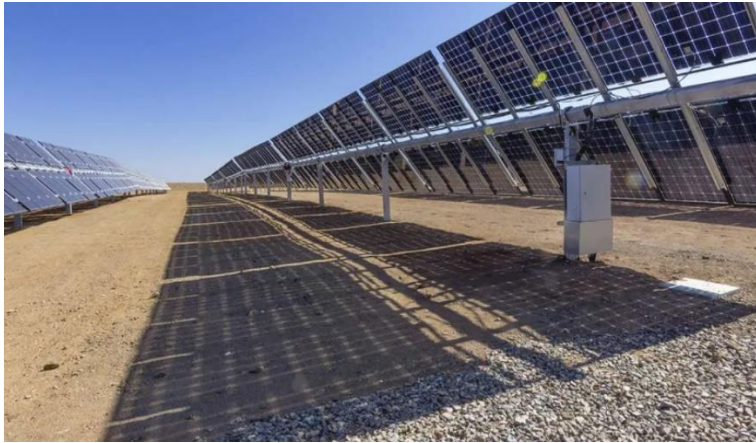
Figure 3: Example of Bi-facial solar panels to be utilised for this project.
