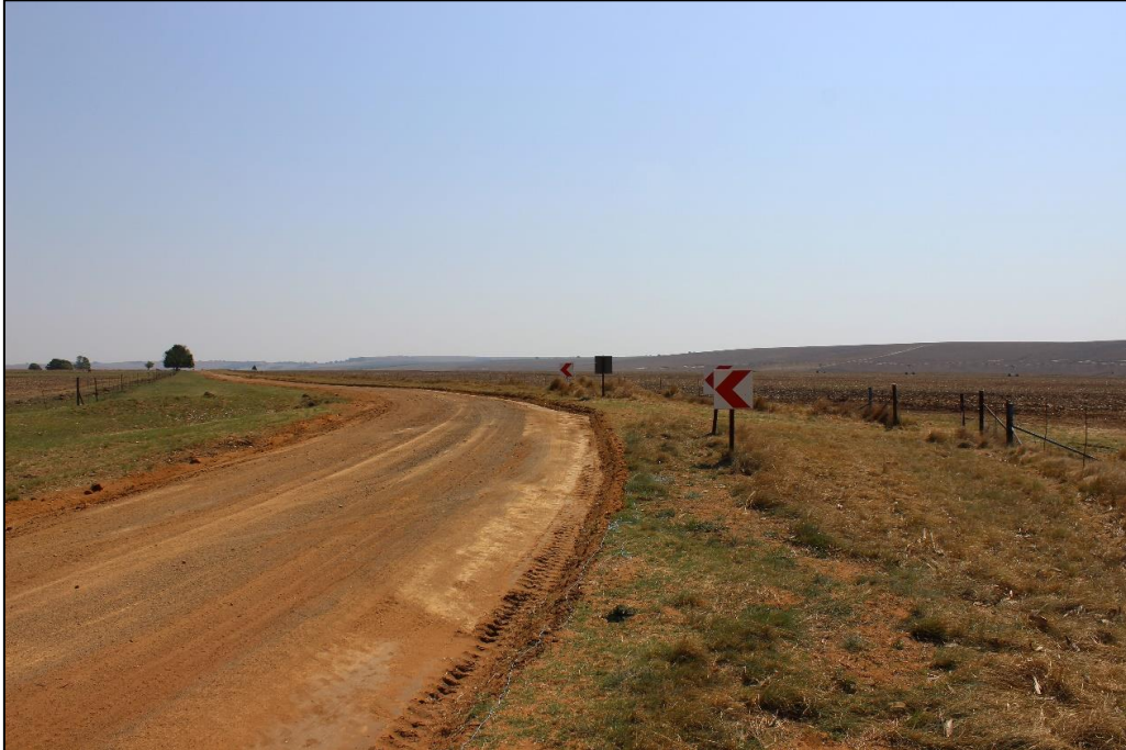
Figure 37: View north from Viewpoint MP3 – Pre-Construction
