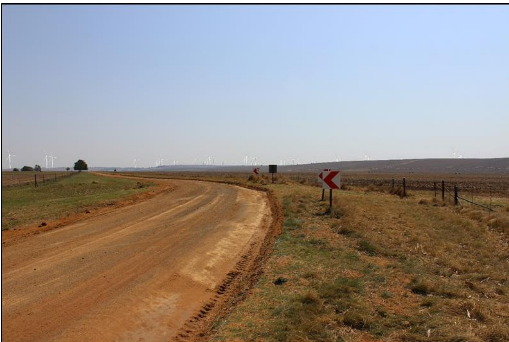
Figure 38: View north from Viewpoint MP3 – Post Construction
