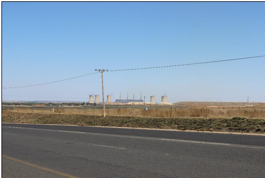
Figure 24: View of Camden Power Station to the west of the N2 national route.
