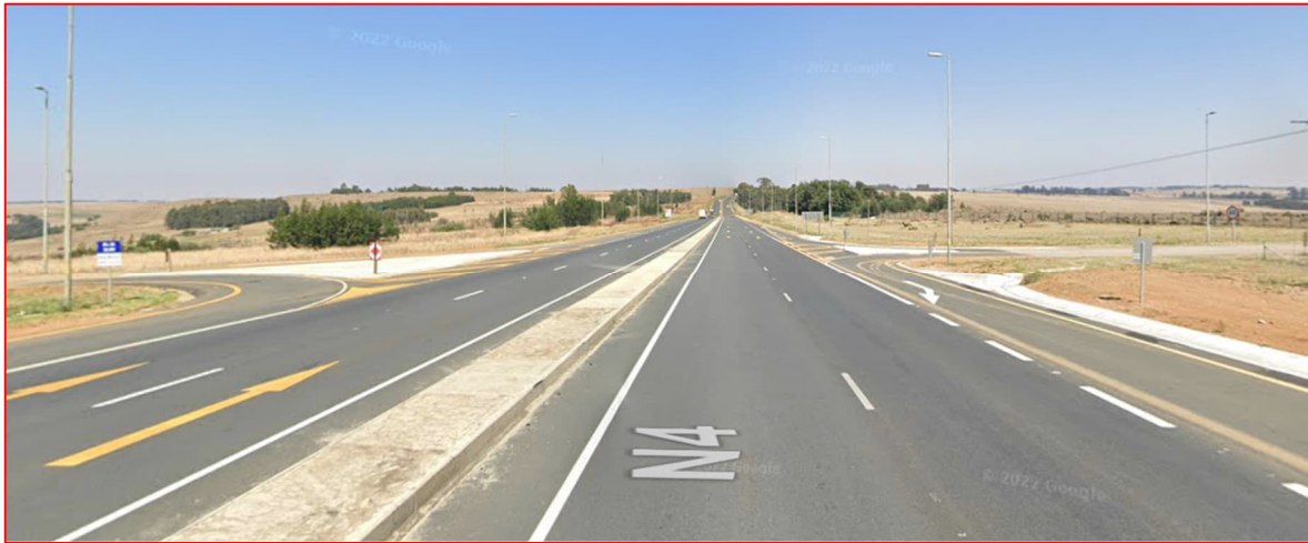
Figure 7-3 N4 westbound approach to the D2524 junction
