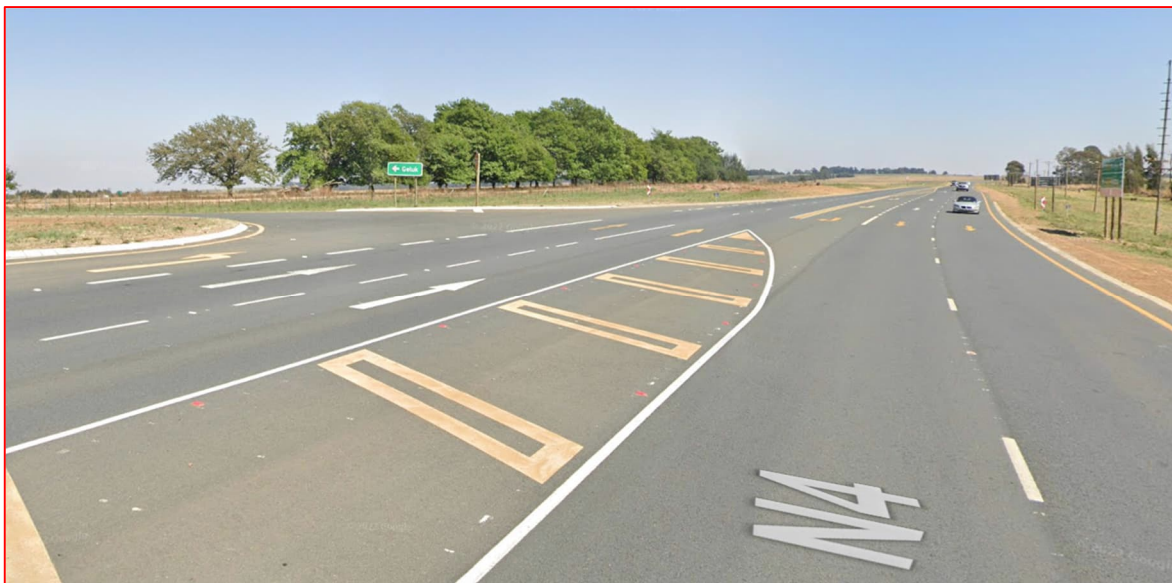
Figure 7-2 N4 westbound approach to the D1039 junction
