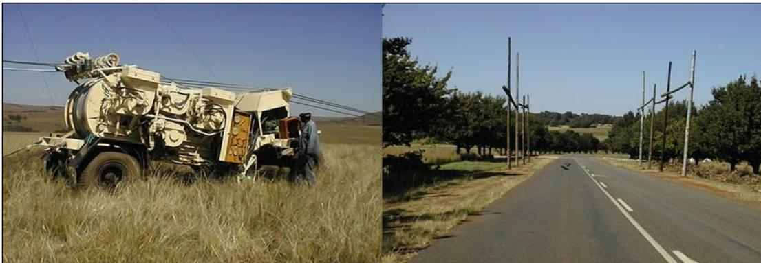
**Figure 1.6: Stringing of conductors (power lines)**
