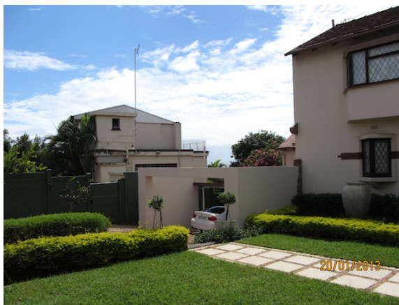
south west view of extension
