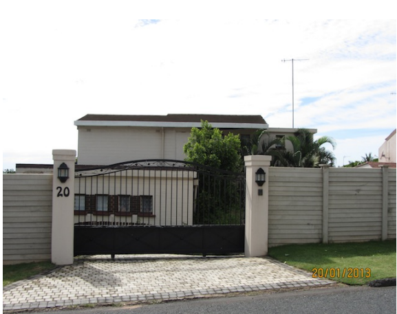
no.20 adjoining property on northern side
