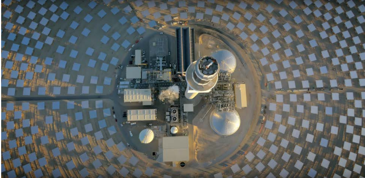
Figure 7 – Near field heliostats are packed densely surrounding the power block
