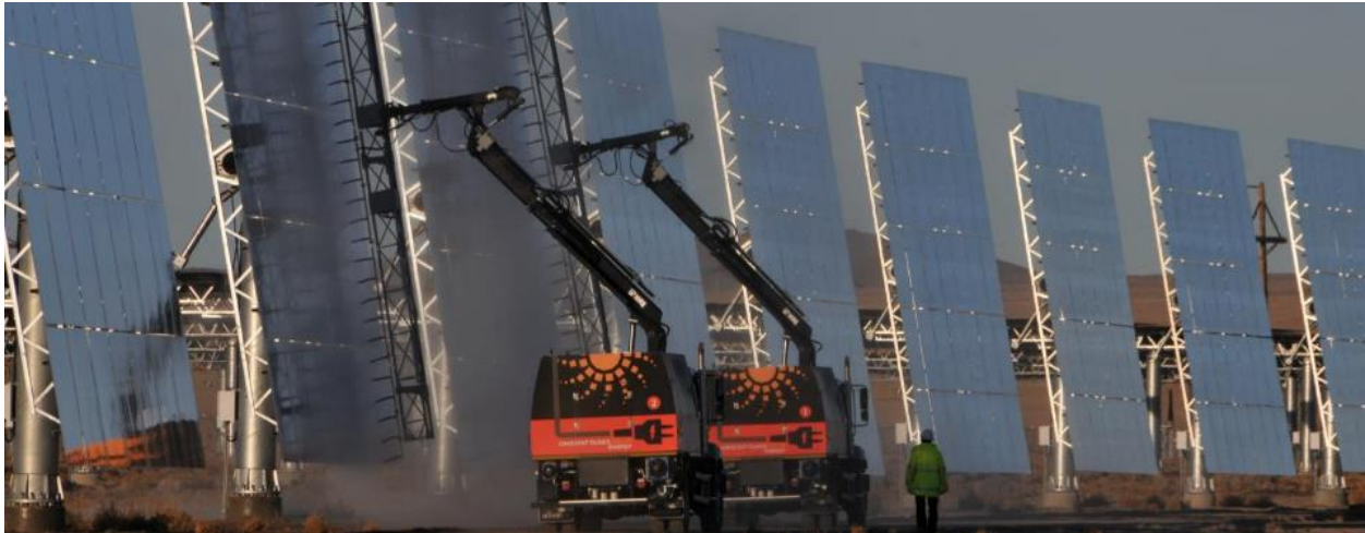
Figure 8 – Wash trucks washing heliostats
