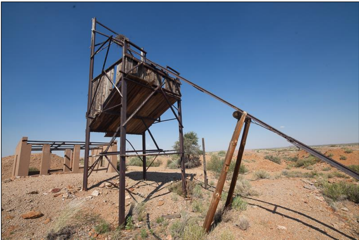
Figure 5 - Headgear at the abandoned tungsten mine on Portion 12 of Dyason's Klip 456. The mine area (about 3,5 ha) will require mitigation should development encroach closer than 50 m
