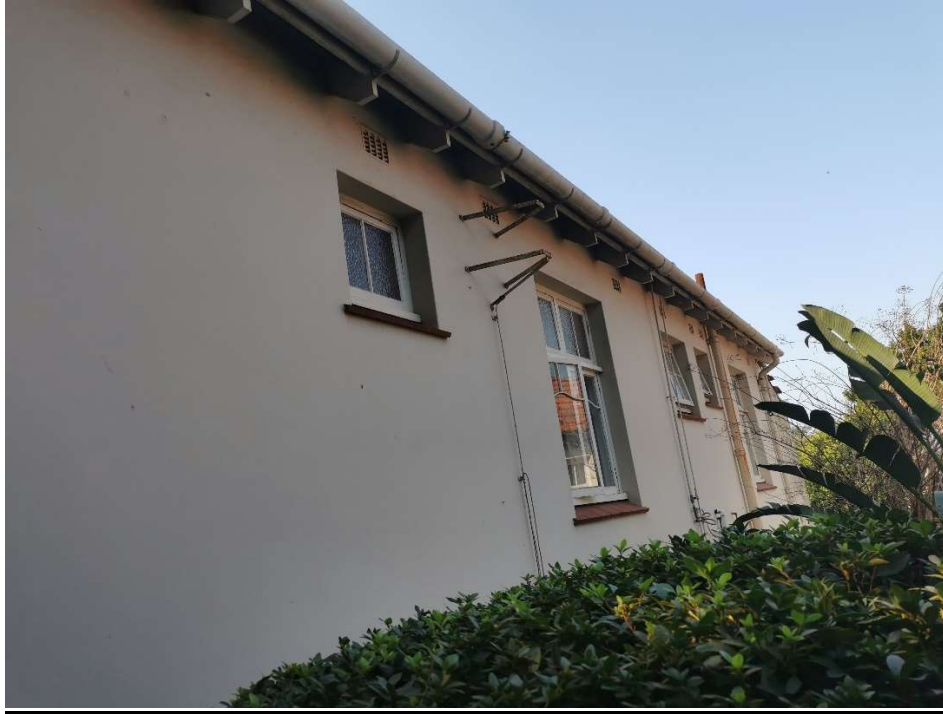
PHOTO 05 – VIEW FROM THE SOUTH WEST (SIDE)
