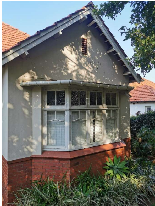
PHOTO 08 – VIEW FROM NORTH WEST (TREMATON DRIVE)
