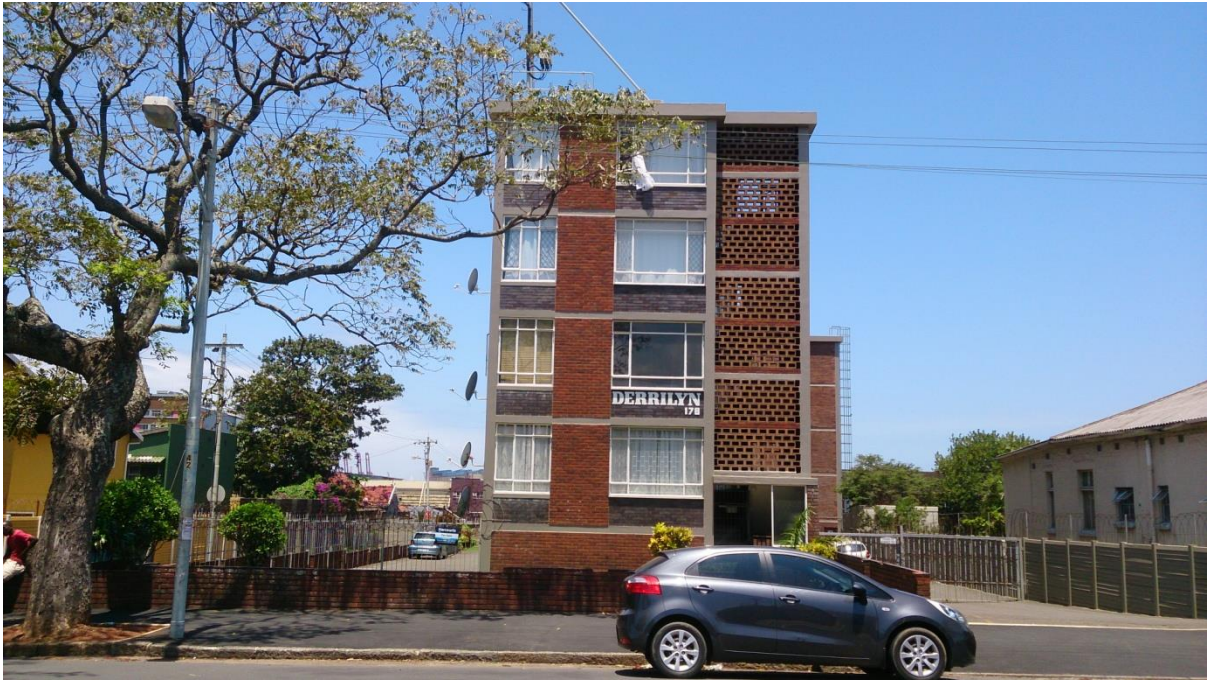
178 ESTHER ROBERTS ROAD – ADJACENT PROPERTY
