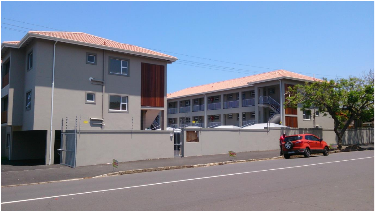
188 ESTHER ROBERTS ROAD – ADJACENT PROPERTY
