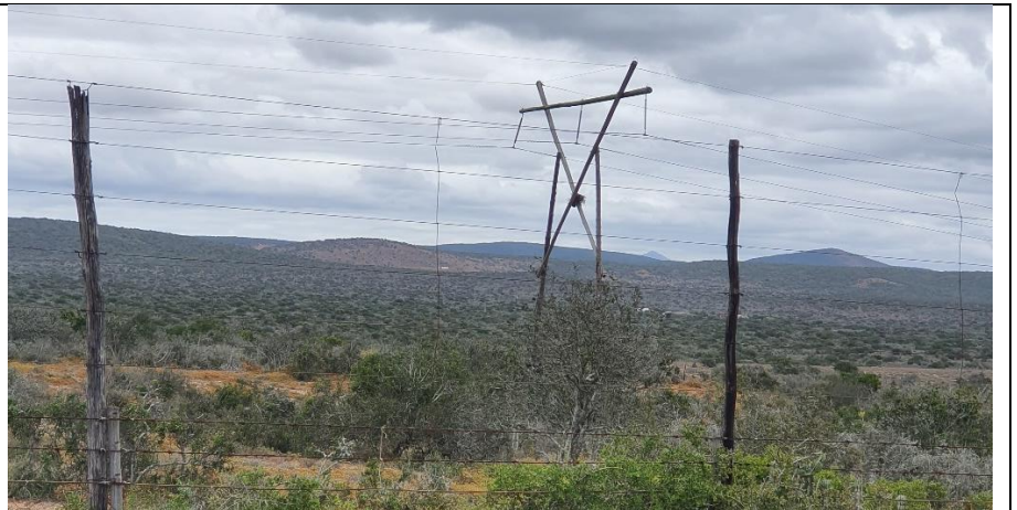
Figure 11: Pylons and powerlines routed adjacent to the R75 road
