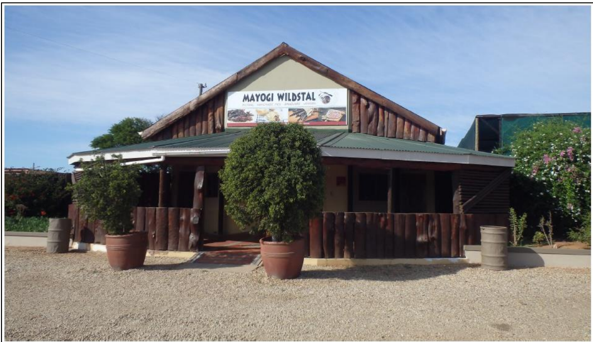
Figure 39: Existing structures located in the south east of the property
