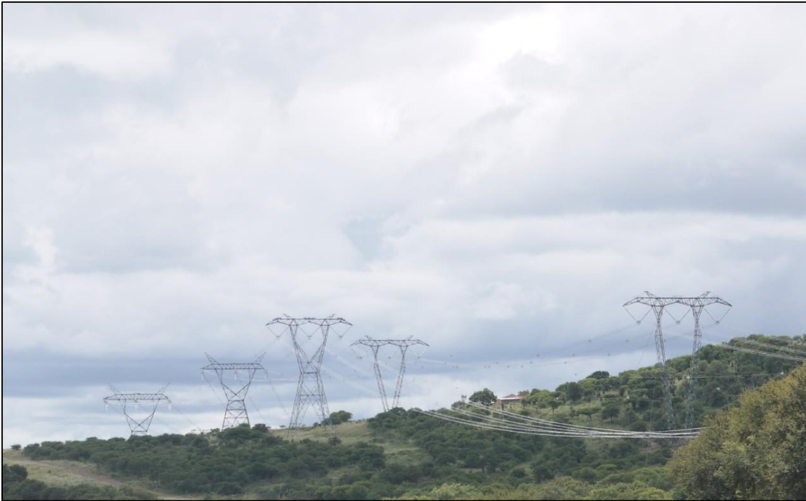
Figure 29: Existing approximately 40m high power lines
