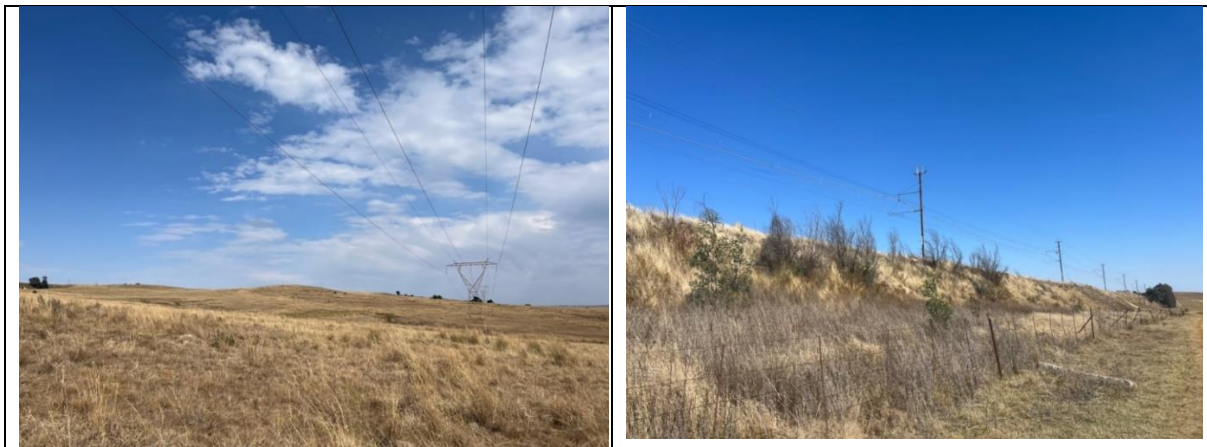
Figure 35: Powerline and railway infrastructure
