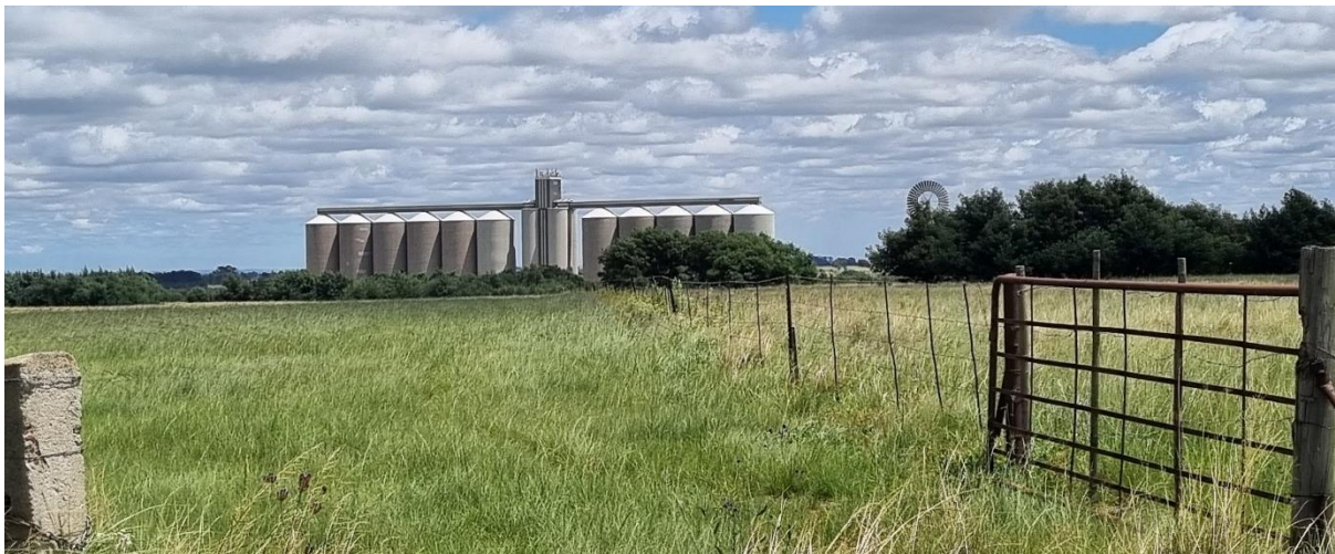
Figure 6: Afagri grain silo
