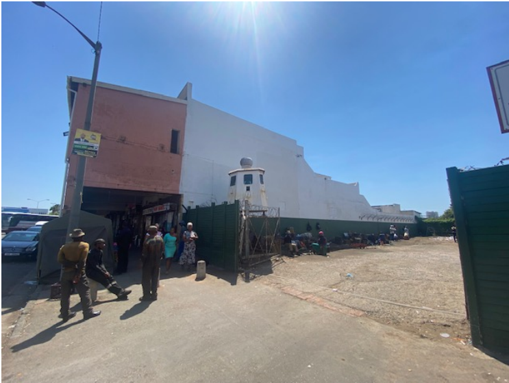
Side View along adjacent site
