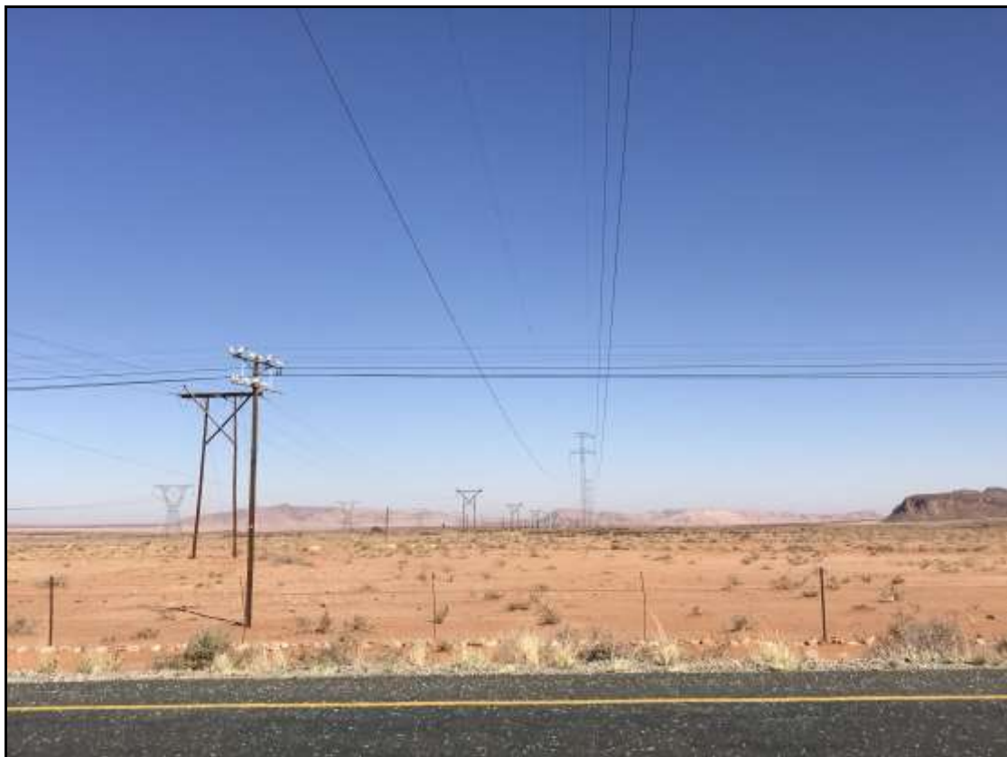
Figure 6: Power lines crossing the access road to Aggeneys near the N14.
