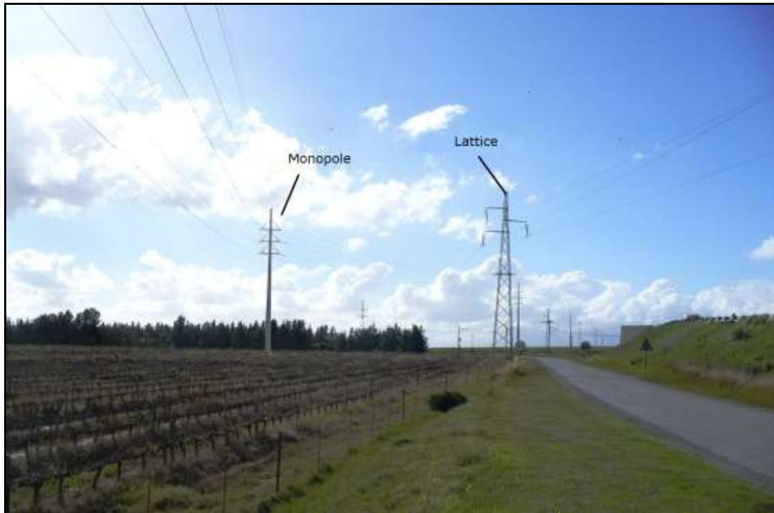
Figure 3: Longer distance view of power line towers.
