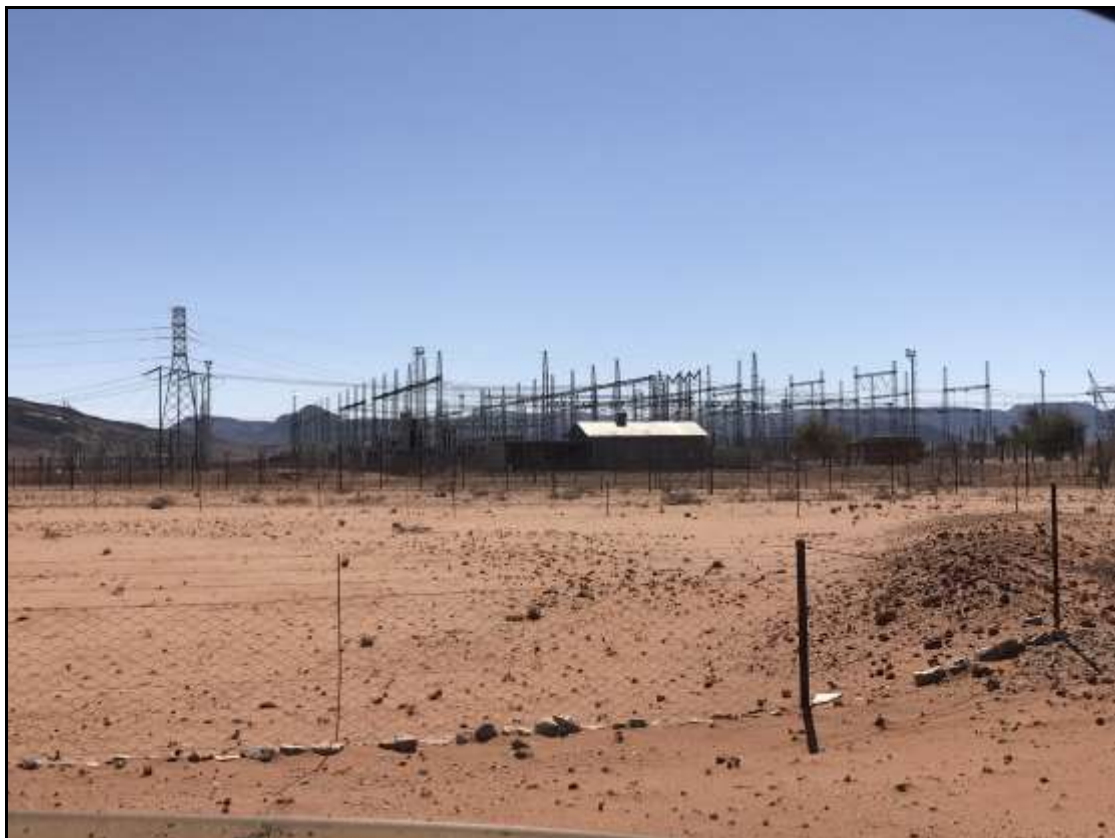
Figure 8: The Aggeneis Substation as seen from the N14.
