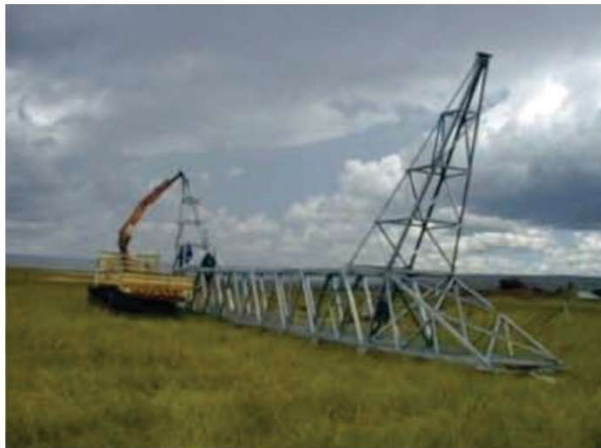
Typical example of crane
