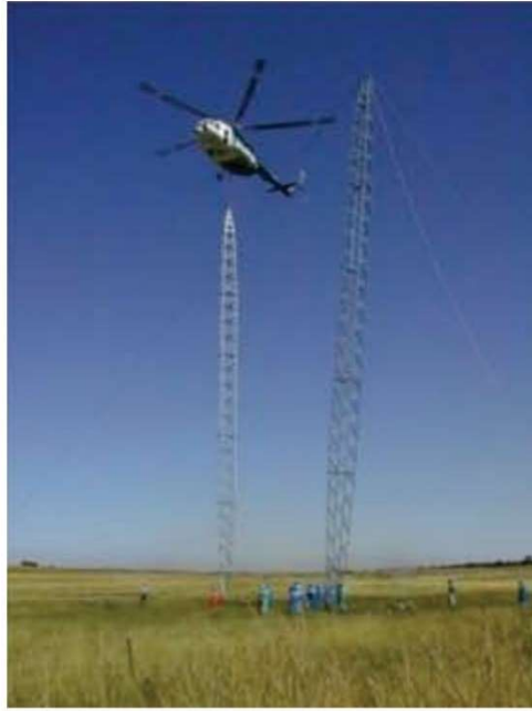
Figure 3: Typical construction equipment
