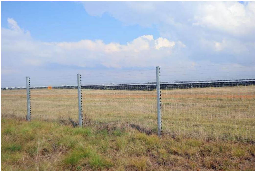
Plate 5, A single axis tracking solar PV project in the North West Province (Bokamoso Solar PV Plant) photographed at approximately mid-day
