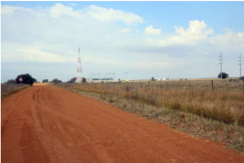
Plate 6, View of on-site substation and exiting overhead power lines via Bus Bars at the substation
