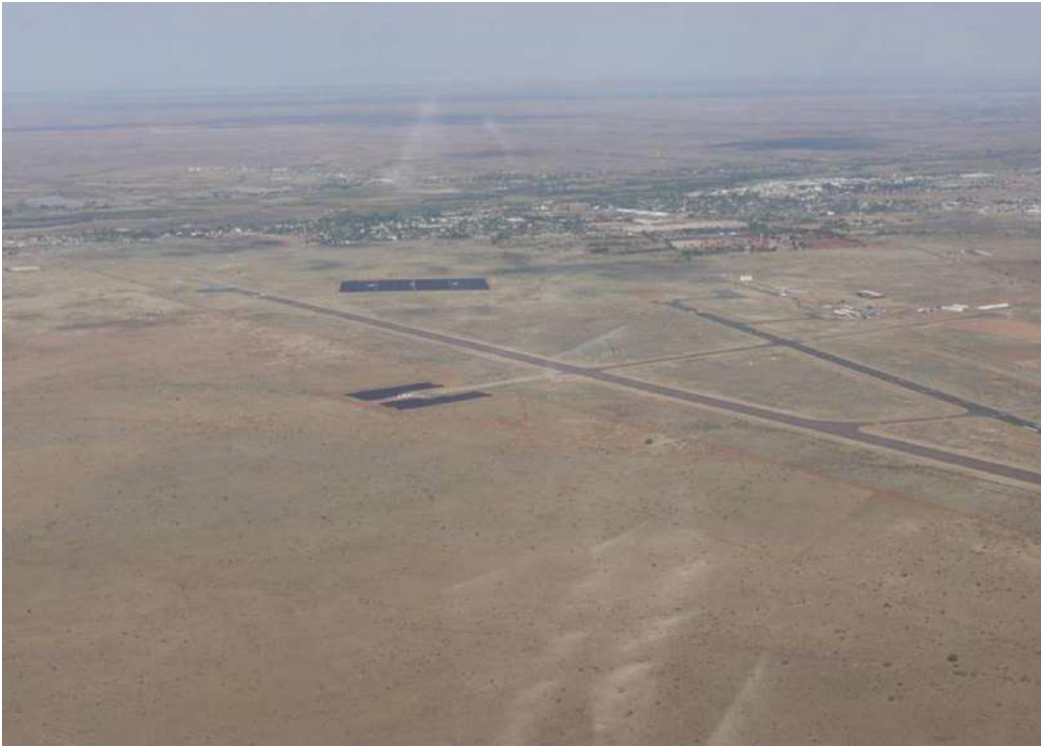
Plate 1, Existing solar arrays at Upington Airport as seen from the air
