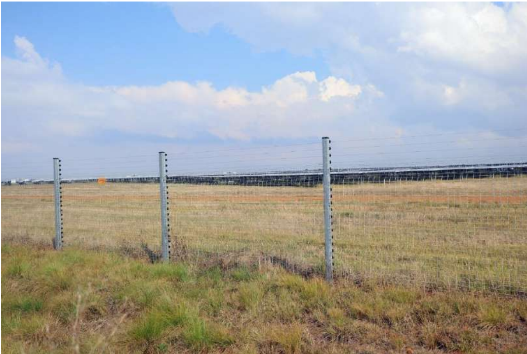
Plate 5, A single axis tracking solar PV project in the North West Province (Bokamoso Solar PV Plant) photographed at approximately mid-day
