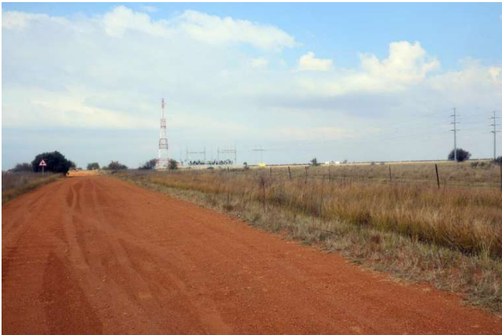
Plate 6, View of on-site substation and exiting overhead power lines via Bus Bars at the substation
