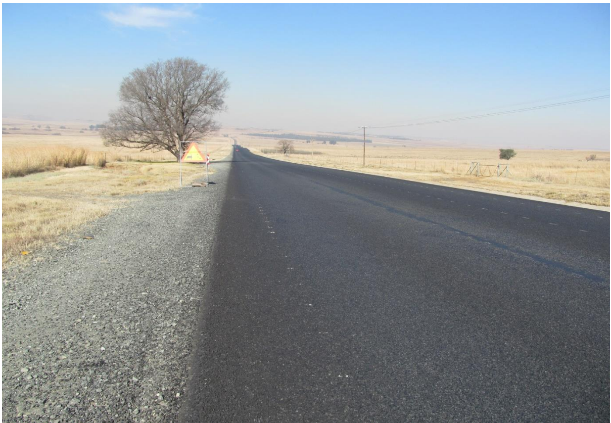
Photo 10: Taken at km 82,4 towards the South East
