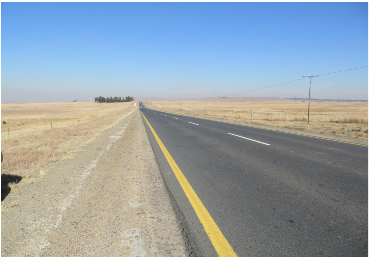
Photo 14: Taken at km 72,4 towards the South East
