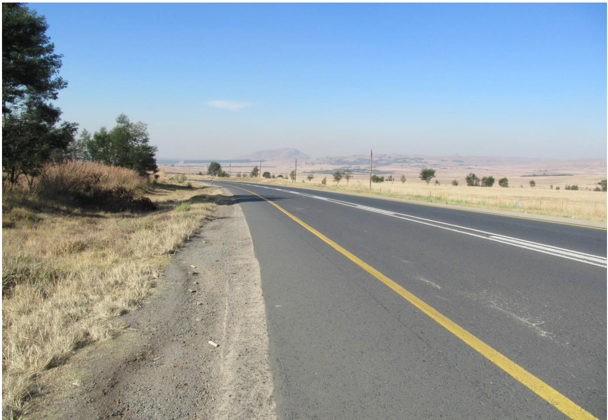
Photo 16: Taken at km 67,4 towards the South East
