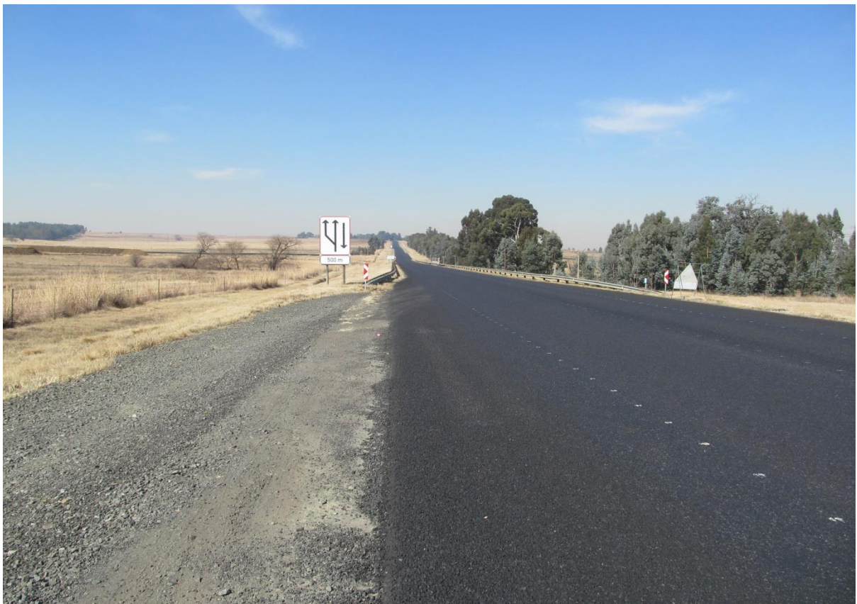
Photo 8: Taken at km 87,4 towards the South East
