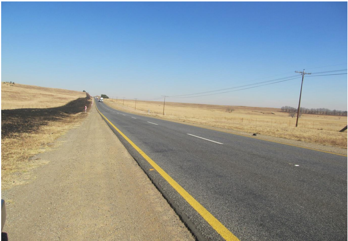
Photo 12: Taken at km 77,4 towards the South East
