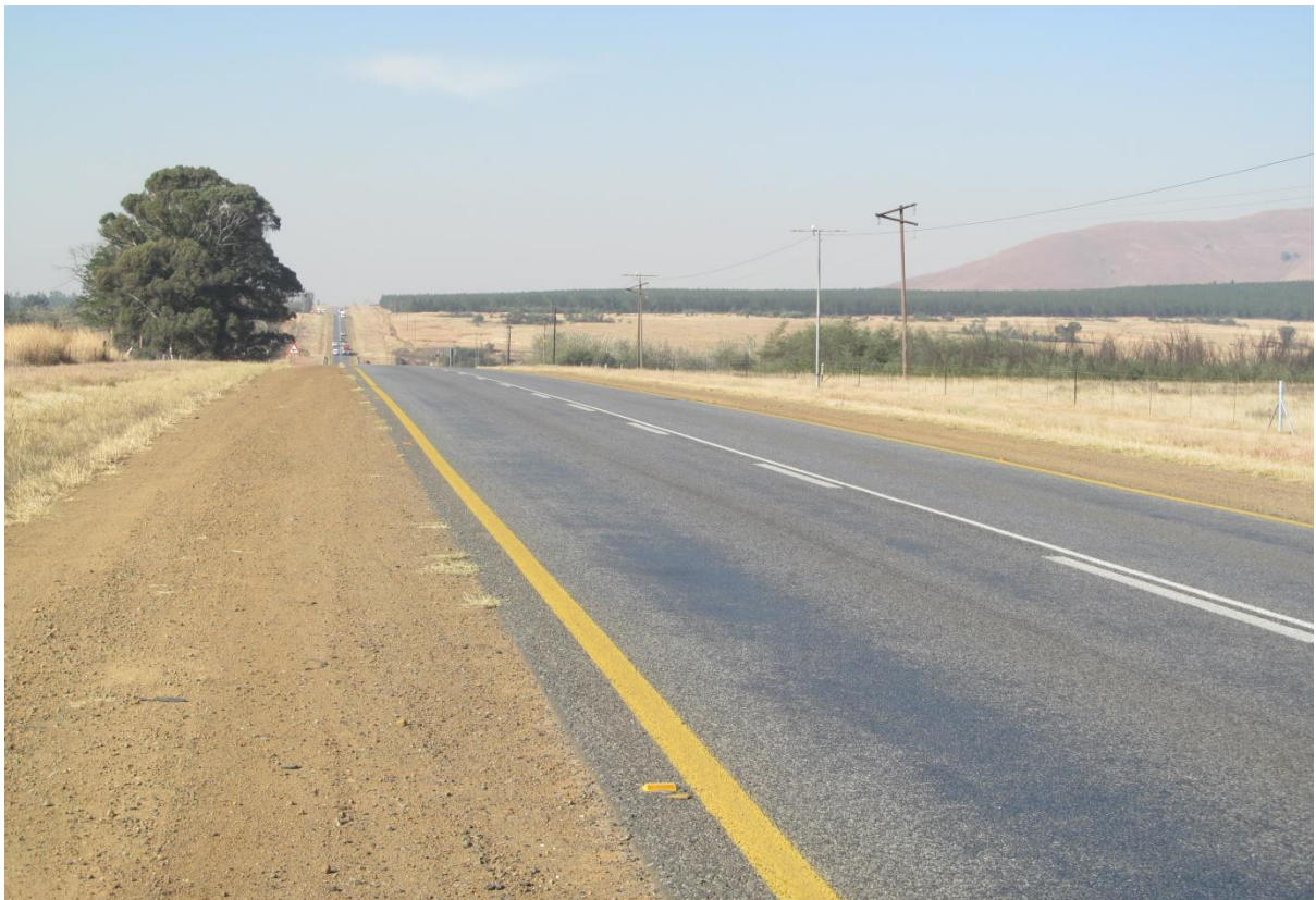
Photo 18: Taken at km 62,4 towards the South East
