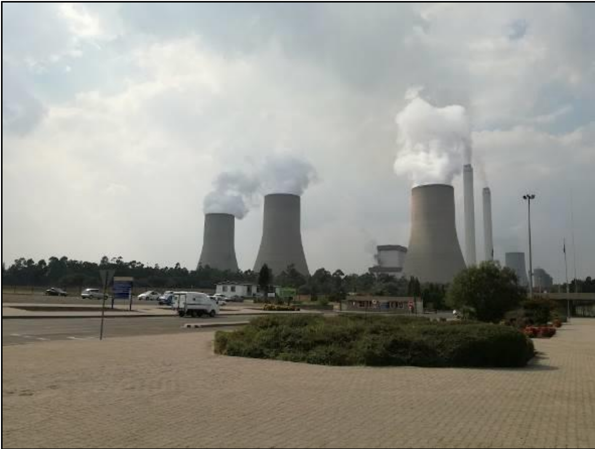
Source: Google Earth Photograph 3.2: Tukuka Power Station
