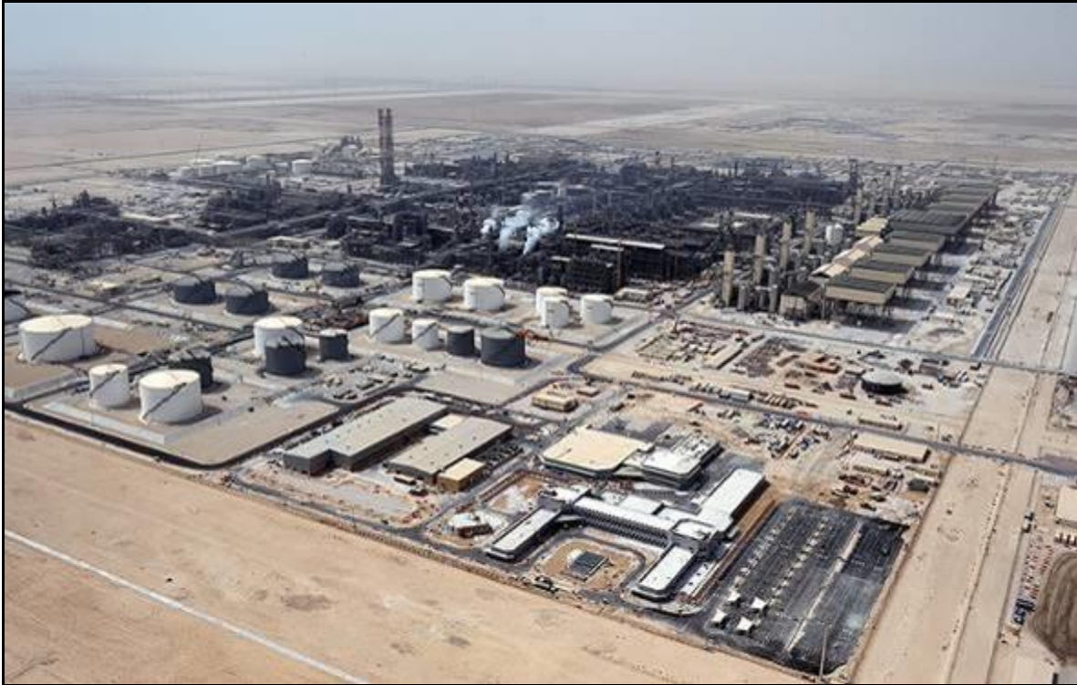
Photograph 3.1: Secunda Sasol Facility
