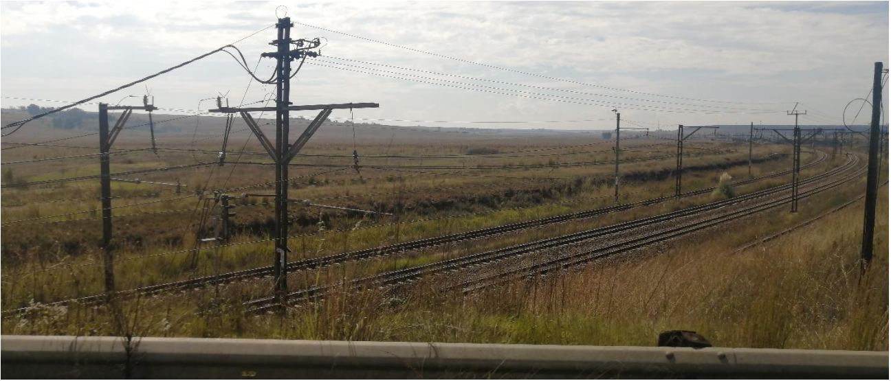
Figure 17: Railway infrastructure used to transport coal in the region
