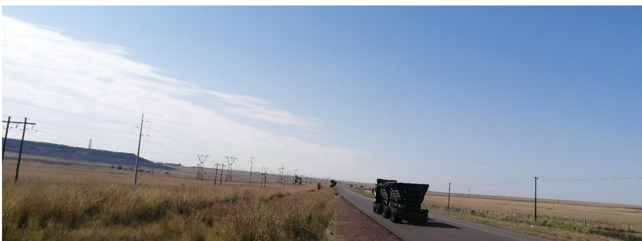
Figure 14: View from the R542 towards the site from the west
