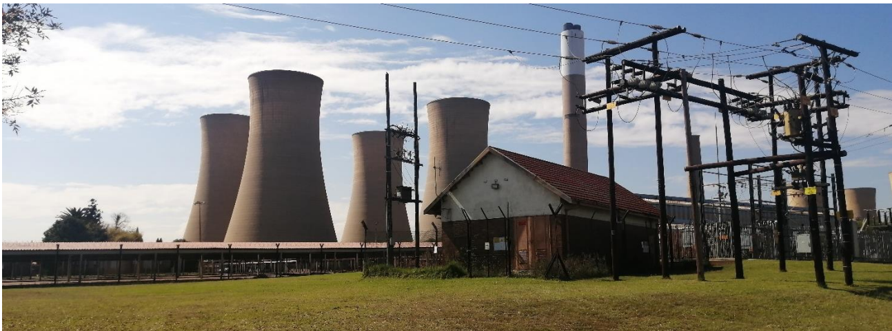
Figure 7: General view of the existing Komati Power Station
