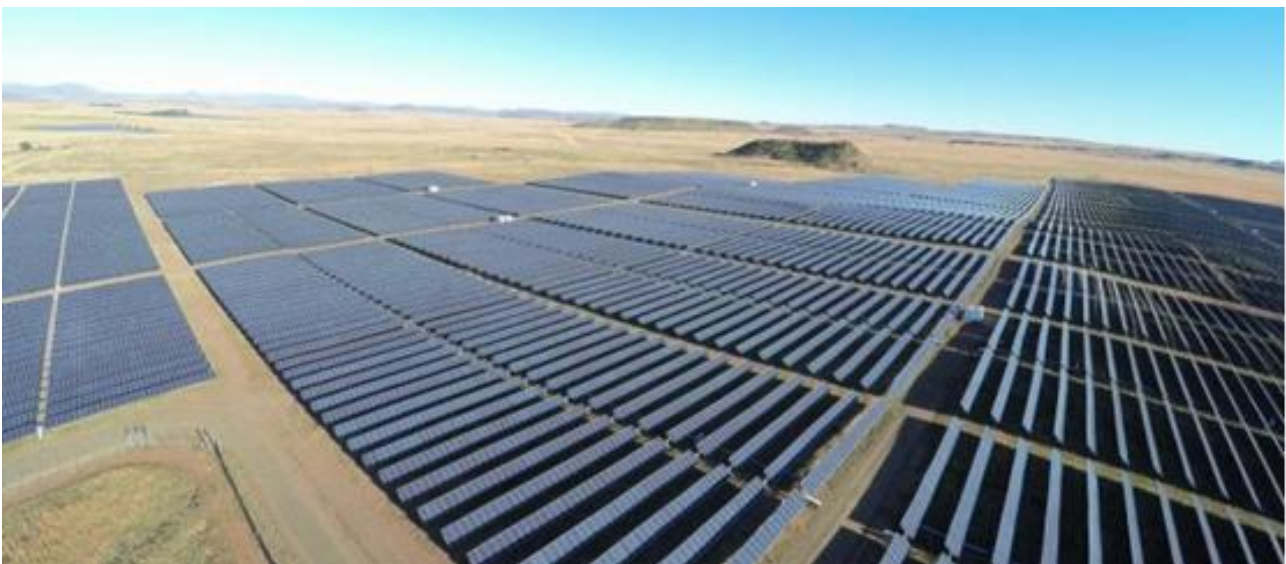
Figure 3: Aerial view of PV arrays. (Photo: Scatec Solar South Africa)
