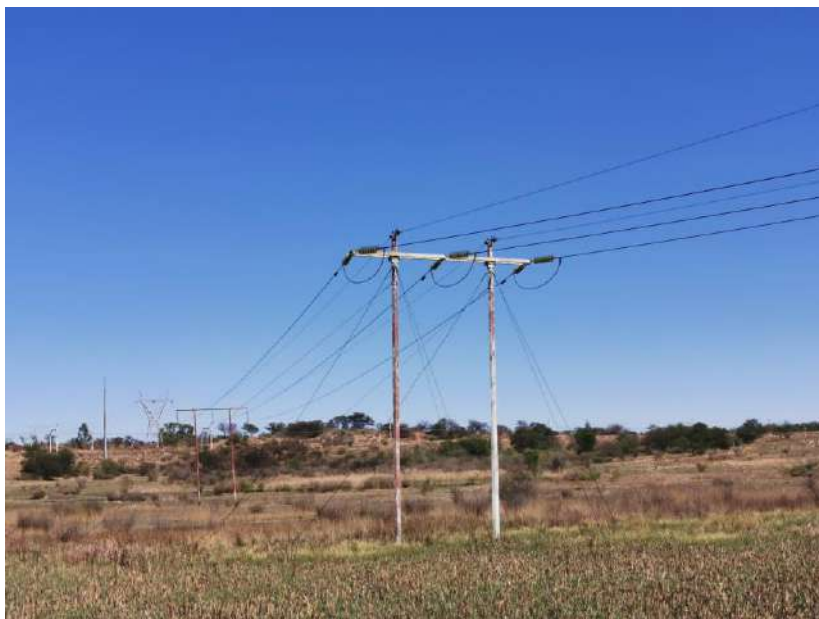
Fig 1.3 – Existing 88kV Incomer to Sonland Milan Substation
