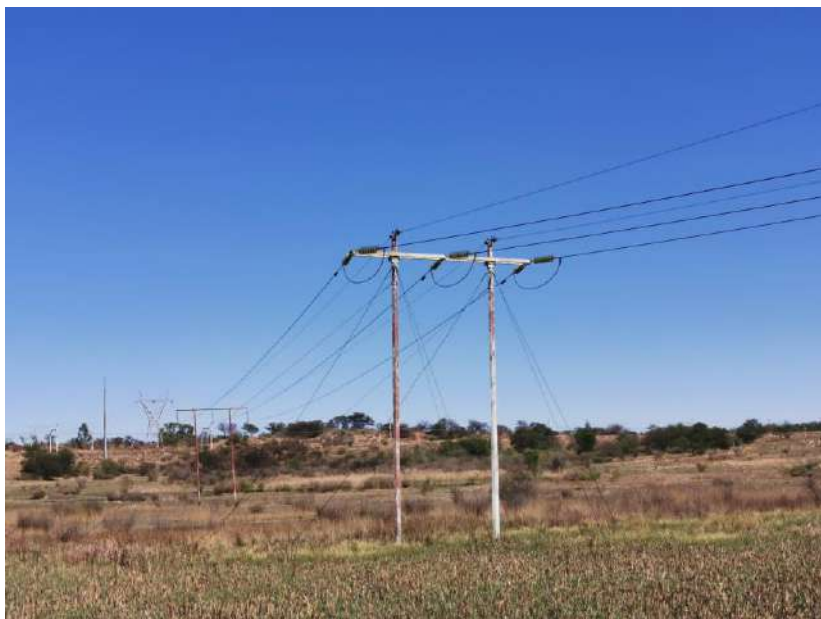
Fig 1.3 – Existing 88kV Incomer to Sonland Milan Substation
