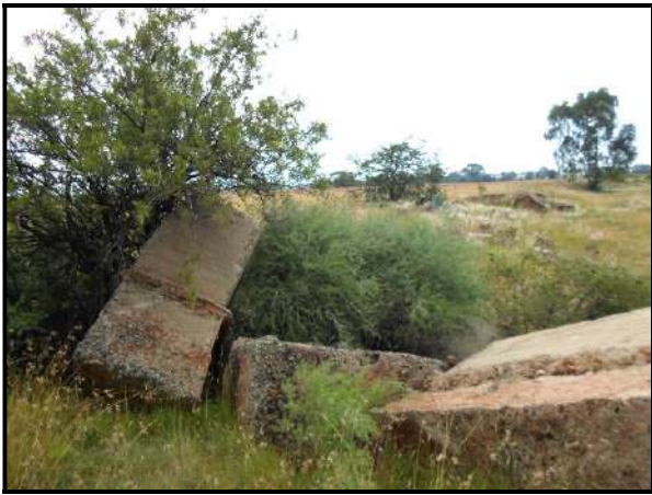
Figure 18. Large foundation slabs.
