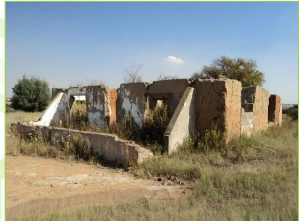
Figure 9.38: Structure W5 seen from the east
