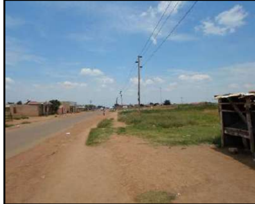
Figure 5. General site conditions - Eastern border.
