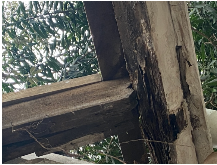
Plate 3.1: Some of the typical wood rot noted in and out of the house during the strip out process.
