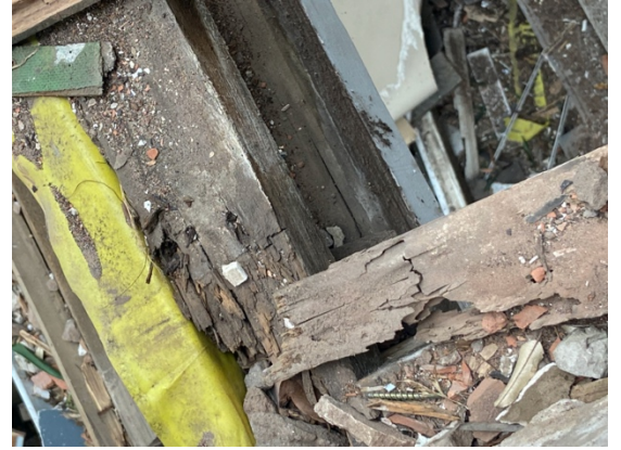
Plate 3.1: Some of the typical wood rot noted in and out of the house during the strip out process.
