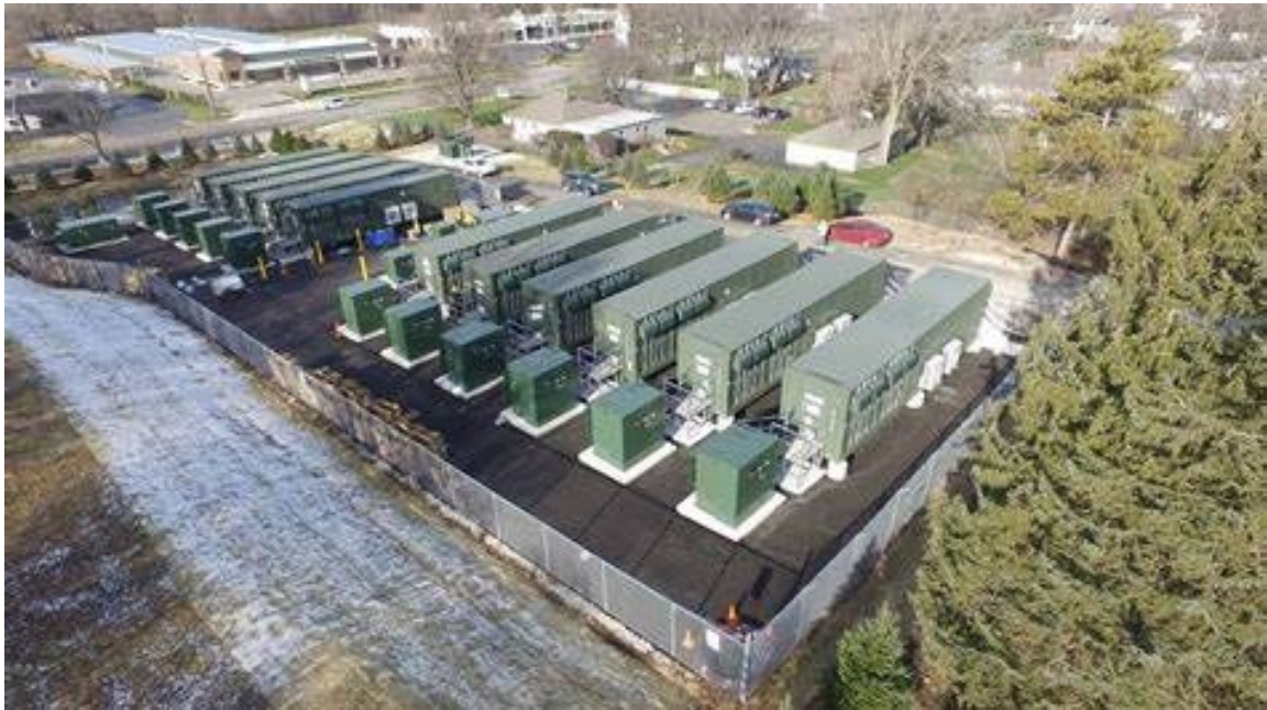
Plate 7 - Typical Battery Energy Storage System
