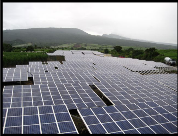
Figure 7 and 8: PV Solar Plant Consisting of Fixed Structures
