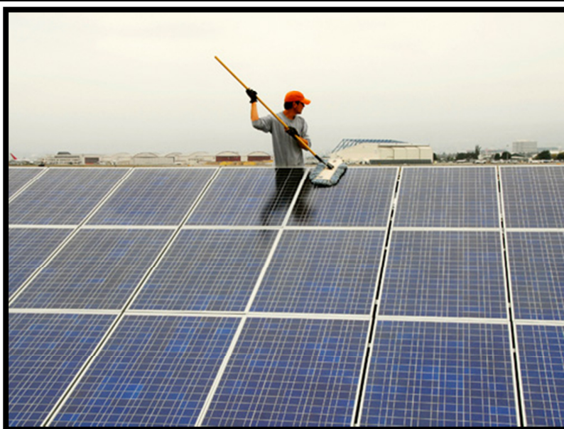
Figure 28: Cleaning PV panels (AE-AMD)
