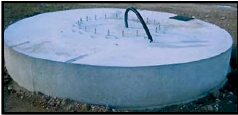
Figure 12: Foundation option for Mecasolar tracker
