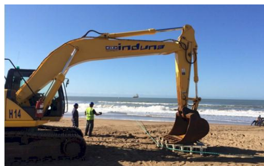
Plate 9 Landing of the cable on shore. Similar works will be undertaken for the landing of the ACE Cable System
