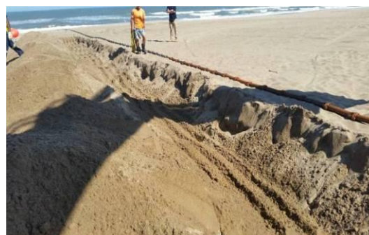
Plate 9 Landing of the cable on shore. Similar works will be undertaken for the landing of the ACE Cable System
