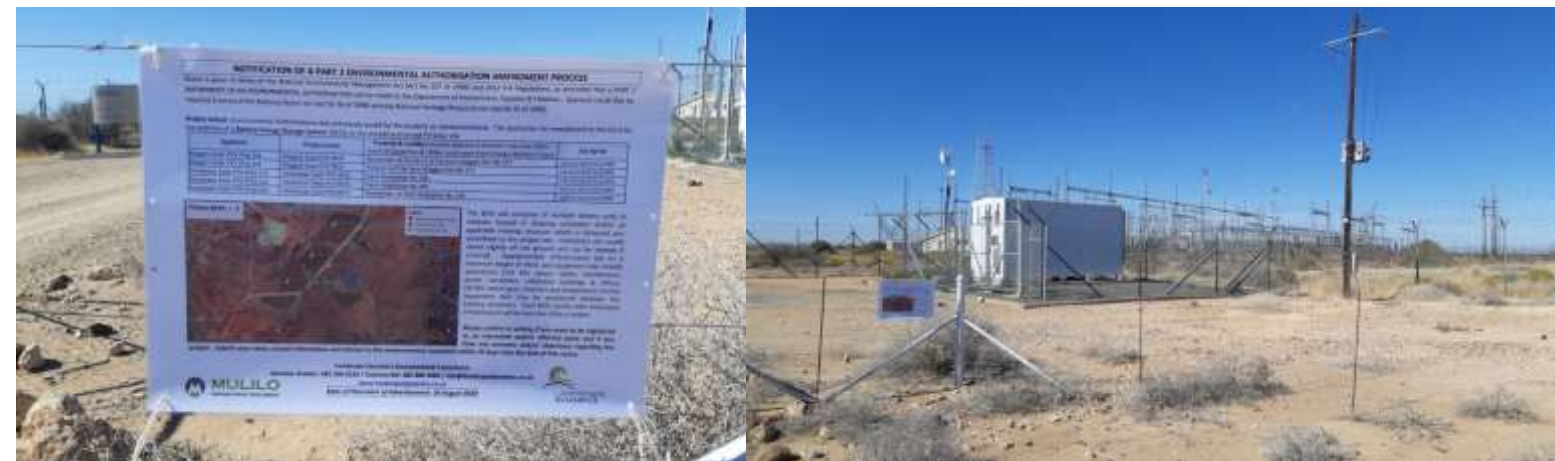
Onsite notice at the Kronos Substation
