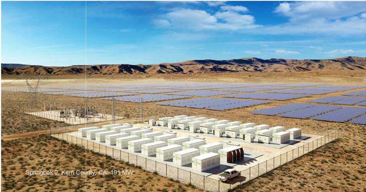
Solar BESS Hybrid Facility in CA USA (Morse, WJ. 2020)
