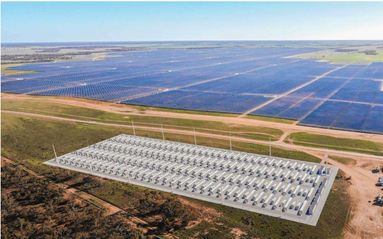
Computer generated image of a similar scale BESS being developed in Australia (Morse,WJ. 2020)
