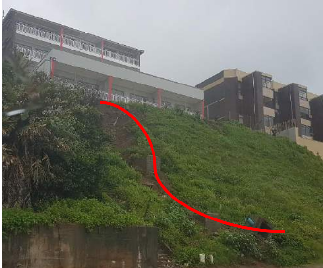
Plate 9: View of the Bank on Seaward Side of the Property.
