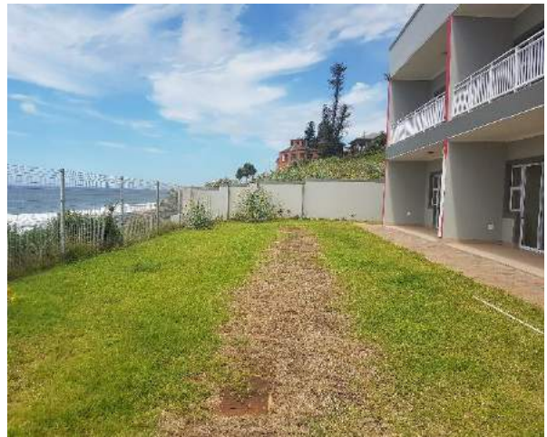
Plate 2: Basement Level View.
