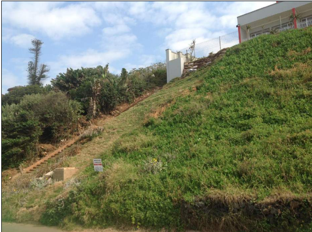
Figure 1: Adjacent Bank Post Re-habilitation.
