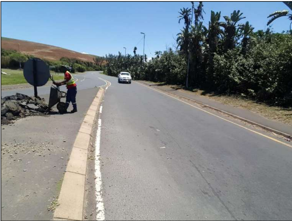
Photo 4: Looking from Casuarina Drive towards the M4 highway south bound.
