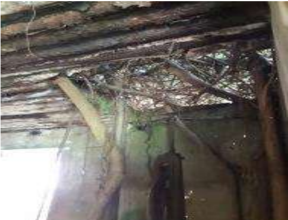
Figure 13: Interior of structure
