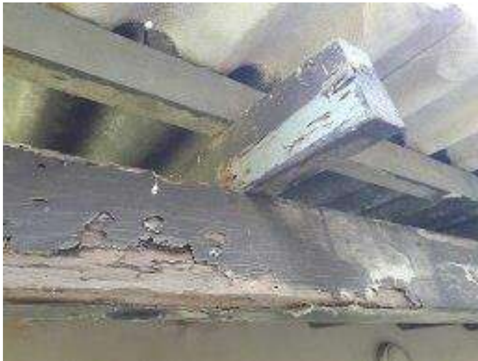
Figure 9: Wooden pillar supporting asbestos roof
