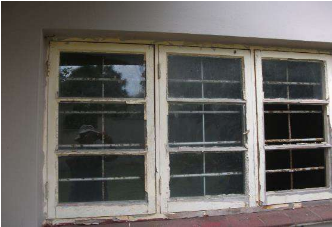
Figure 7: Wooden window frames
